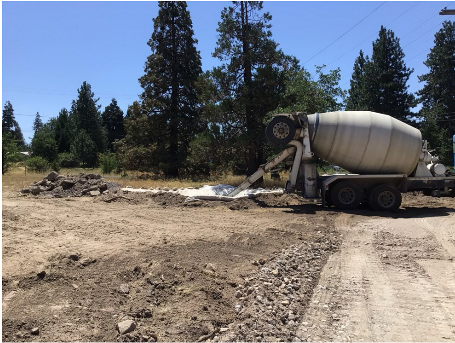
Photo 3: Completed installation of concrete truck washout
