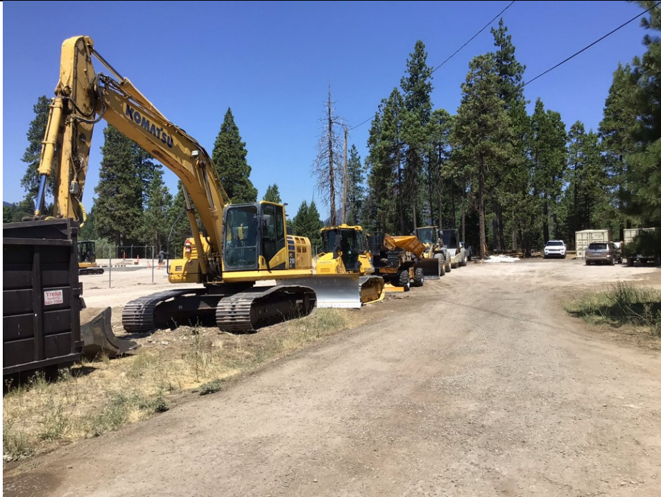
Photo 1: Staging of delivered equipment
