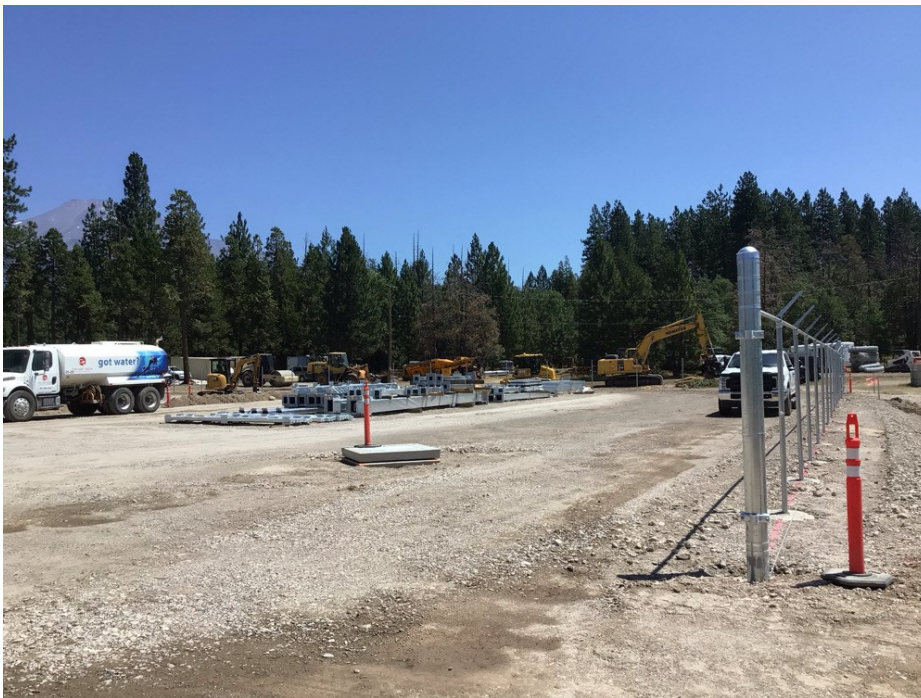
Photo 2: Installed fencing by the constructed substation platform and other excavation work
