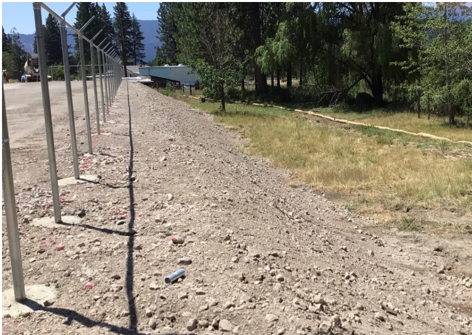
Photo 4: SWPPP erosion control BMPs (fiber rolls) in good condition along NW project boundary in accordance with APM WQ-1
