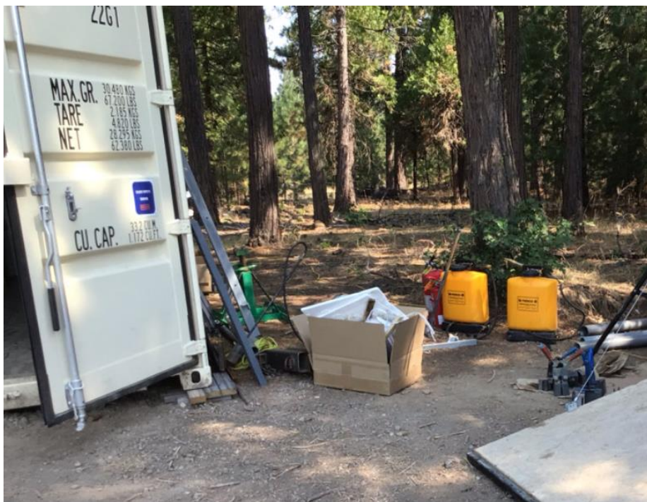
Photo 4: Fire Equipment was staged on site in accordance with the project's Fire Plan (MM HAZ-2).
