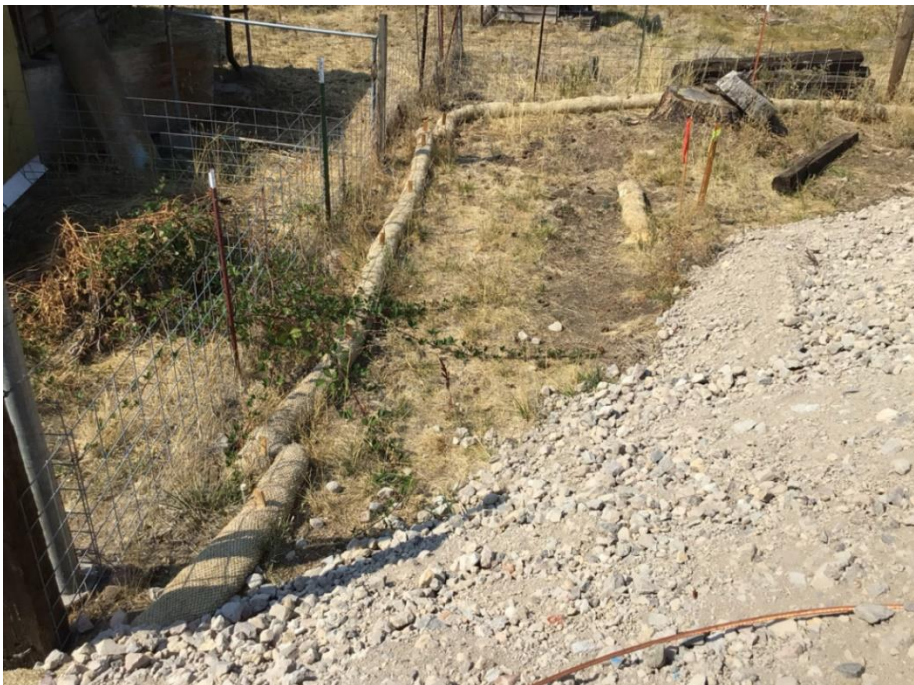
Photo 2: SWPPP erosion control BMPs (fiber rolls) were observed in good condition along the project boundary in accordance with APM WQ-1.
