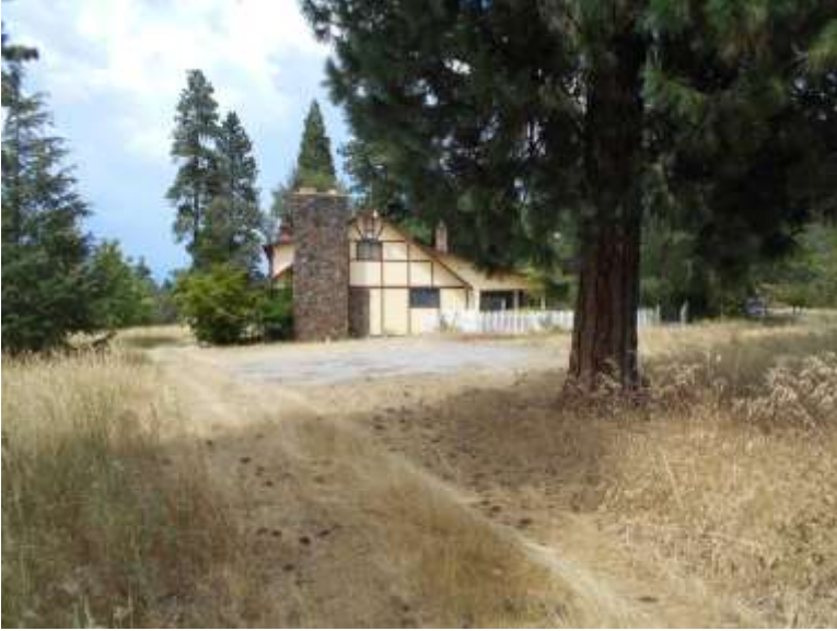
Photo 5. View facing north of 504 South Old Stage Road.
