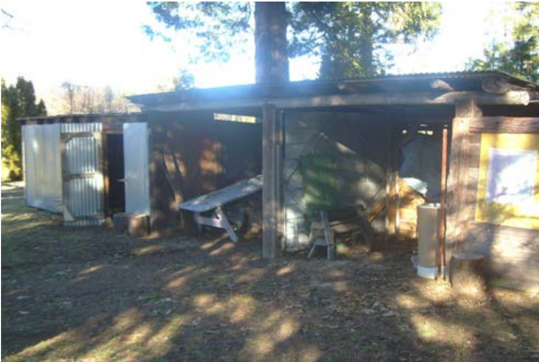
Photo 6. View of the storage shed.
