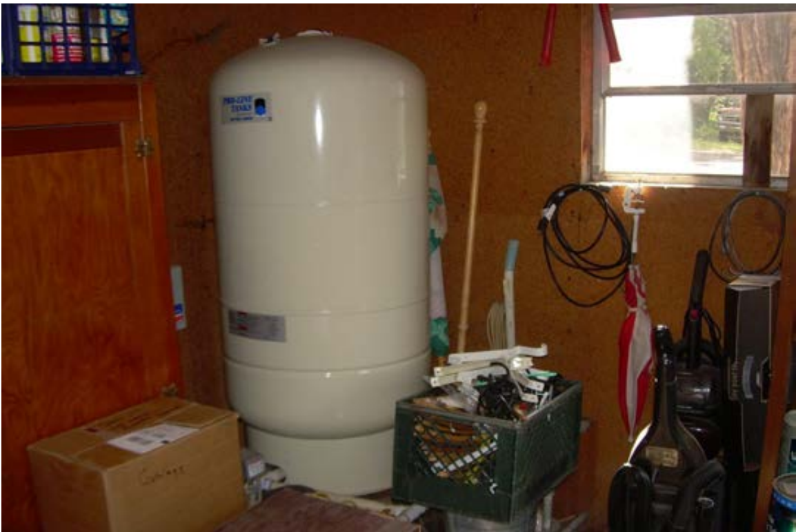
Photo 6. Interior view of the well shed.
