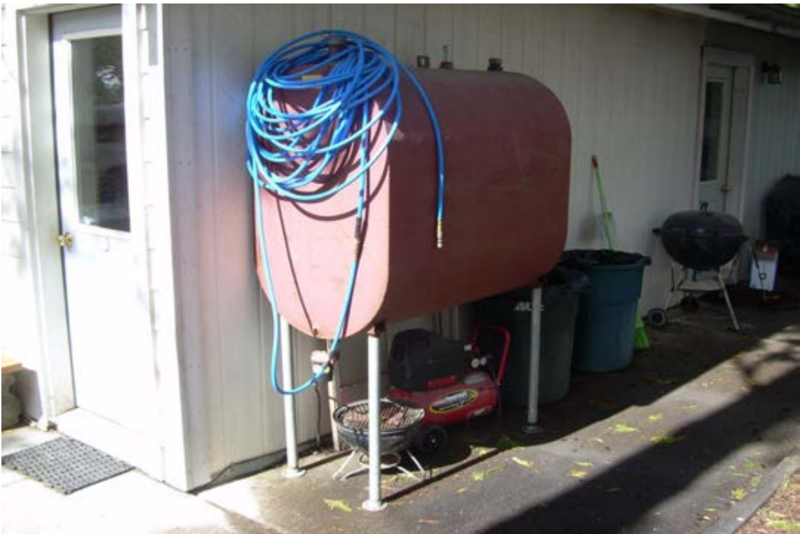
Photo 4. View of the heating oil AST located adjacent to the residence.
