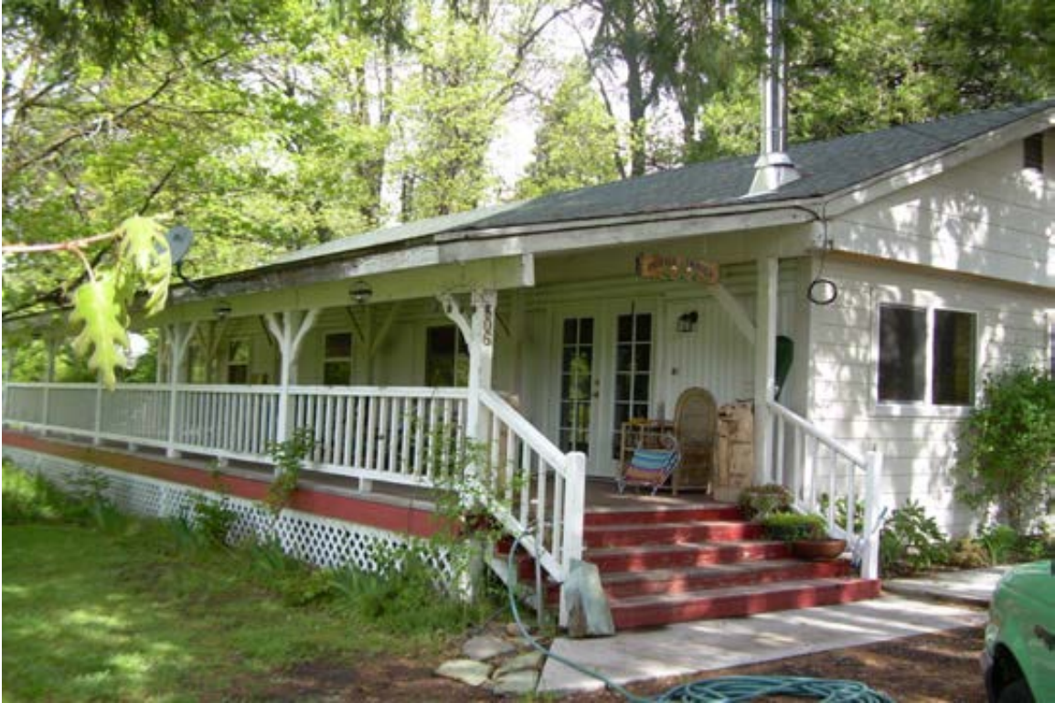
Photo 1. View of the residence located on the property.
