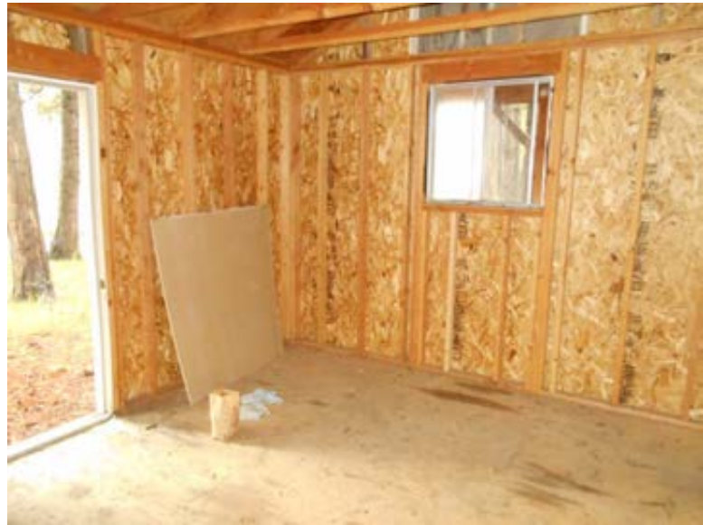
Photo 8. Interior view of the storage shed at 506 South Old Stage Road.
