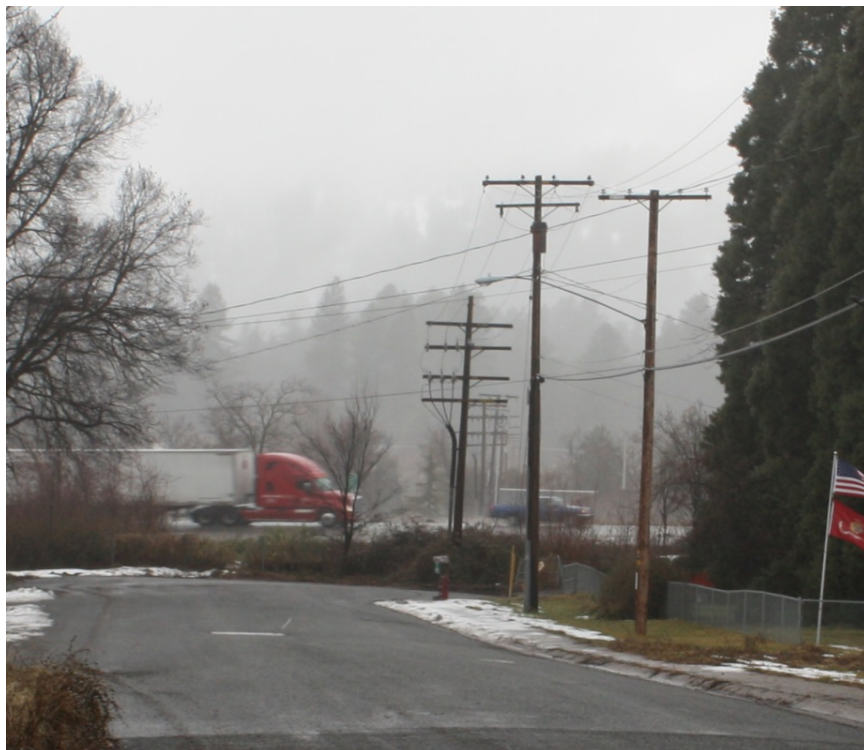
Figure 3: Existing Transmission East of I-5
