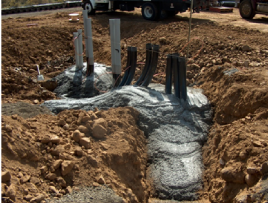
Figure 2—FTB Around Conduits Prior to Concrete Foundation Placement
