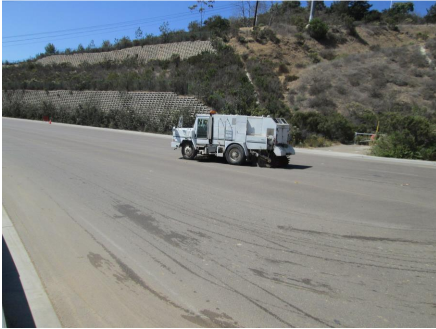
Photo 3: A street sweeper is being utilized along Mira Sorrento Place to minimize trac-out along paved roadway surfaces.
