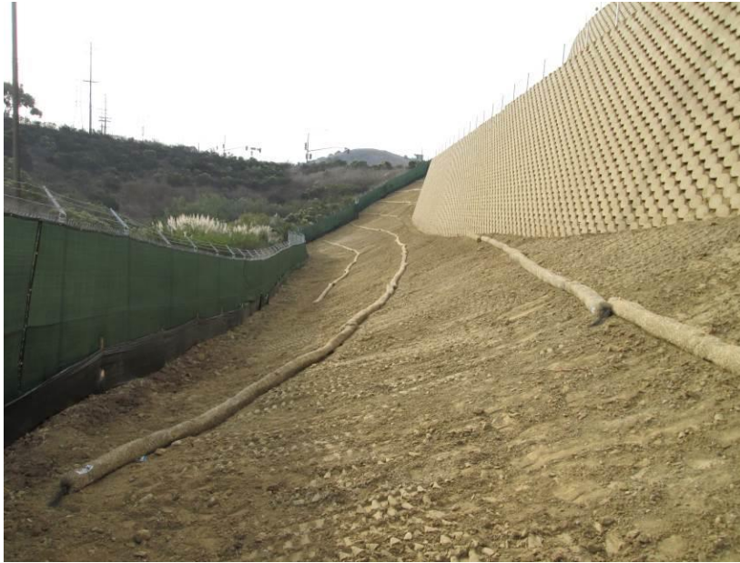
Photo 3: In accordance with APM-HYD-1, silt fencing remains intact along the eastern project site perimeter, and a series of straw wattles have been installed along the adjacent slope.
