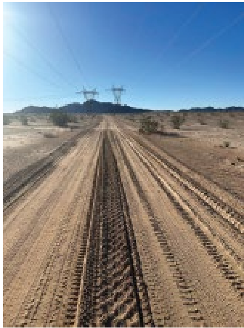
Photo 2: Crews are continually spraying roads to prevent fugitive dust in accordance with BMP-BIO-34.
