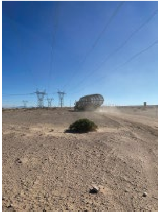
Photo 3: Materials delivery utilizing approved access road.
