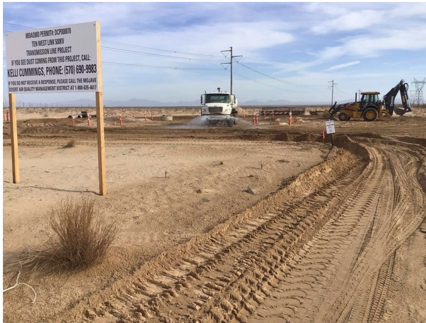
Photo 2: Crews are continually spraying roads to prevent fugitive dust in accordance with BMP-BIO-34.
