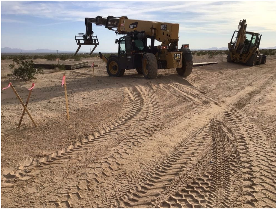
Photo 3: Crews placing timber mats over underground gas line.
