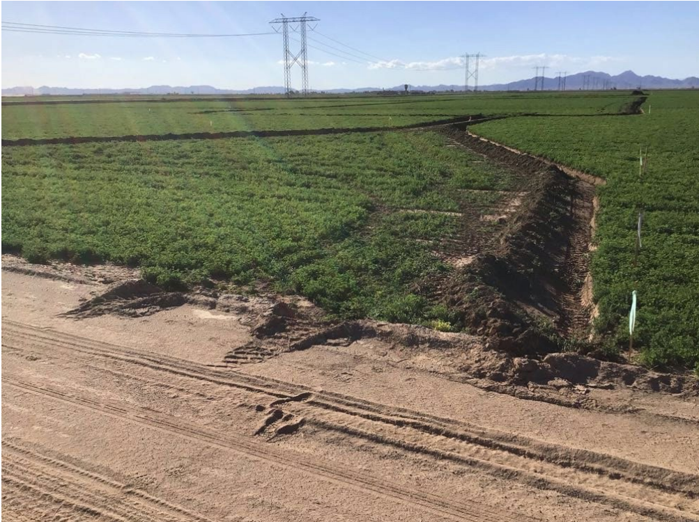
Photo 5: LOD outline trenched.
