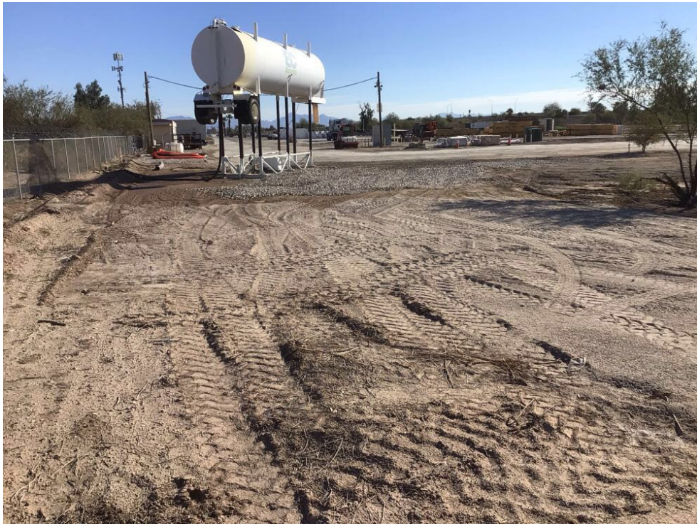
Photo 4: No pooling at the water fill station.
