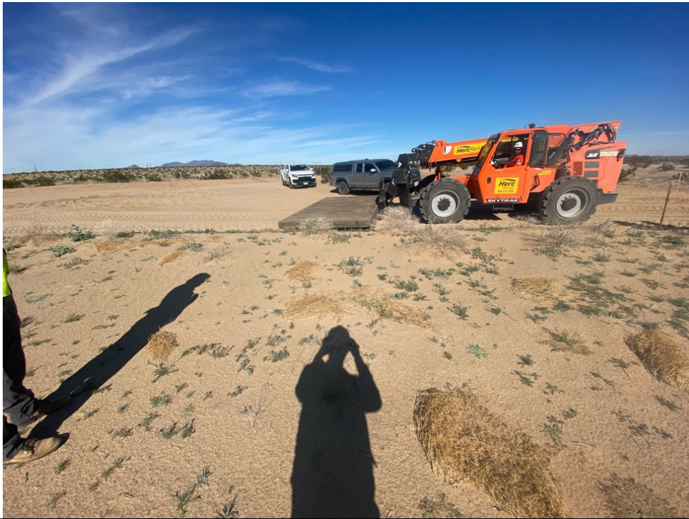
Photo 3: Timber mat installation occurring near the southern weed wash station.
