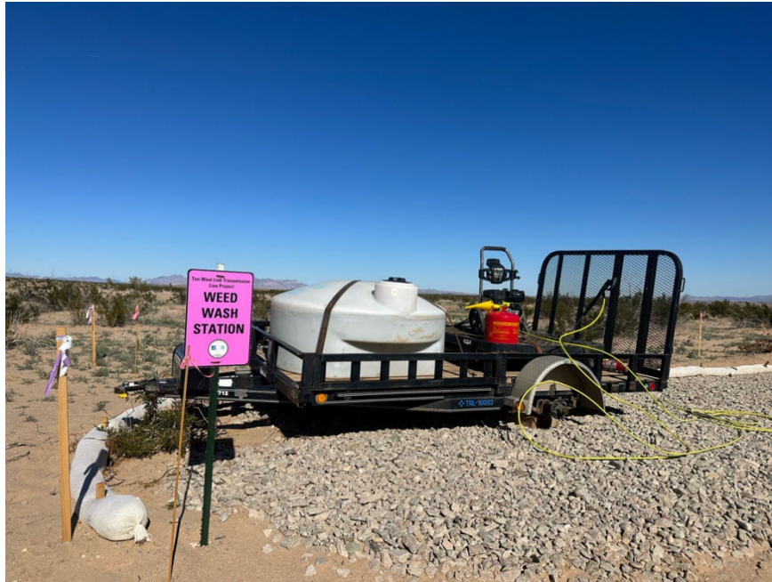
Photo 1: Weed wash station present in accordance with APM-BIO-12.
