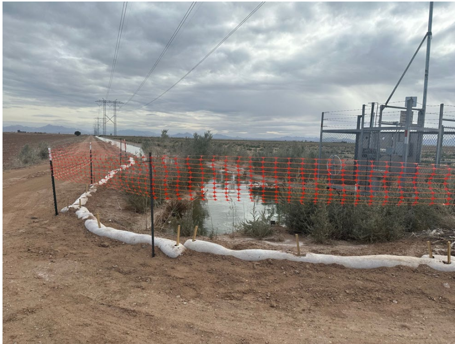
Photo 2 Straw waddles functional near tower 382 in accordance with APM WQ-01.
