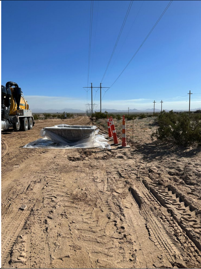
Photo 3: Designated concrete washout station.
