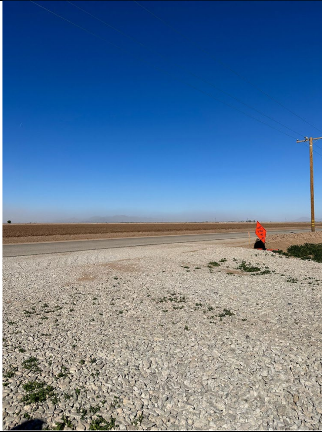
Photo 4: Gravel installed to reduce track out.
