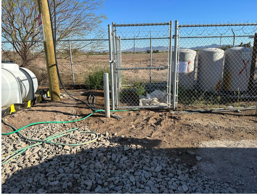
Photo 1: No pooling water in the laydown yard on Hobson way and HWY 78 in accordance with BMP BIO-34.
