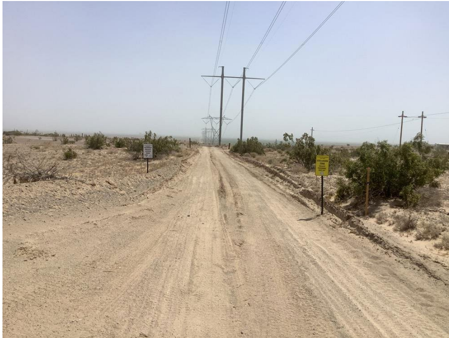
Photo 4: Proper signage installed to avoid exclusion zones.
