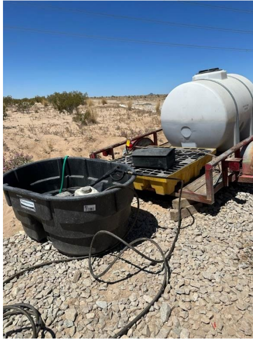
Photo 3: Fire extinguisher present at wash station and power washer contained inside secondary containment.
