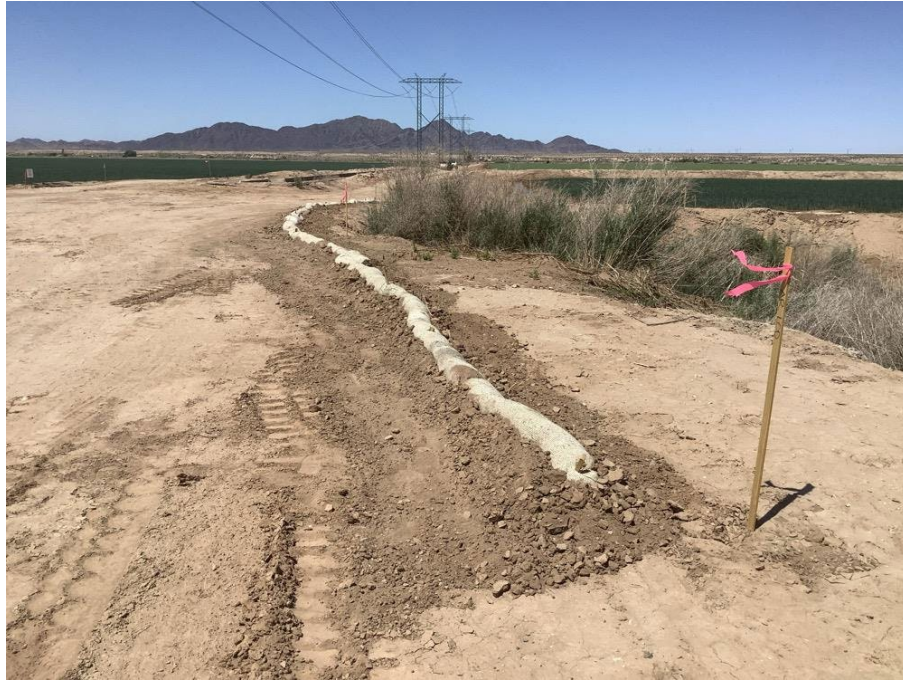
Photo 5: BIO-10 BMP installation of straw wattles site 374.
