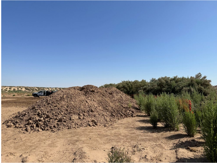
Photo 3: Spoil piles inside LOD in accordance with AMP-BIO-03.
