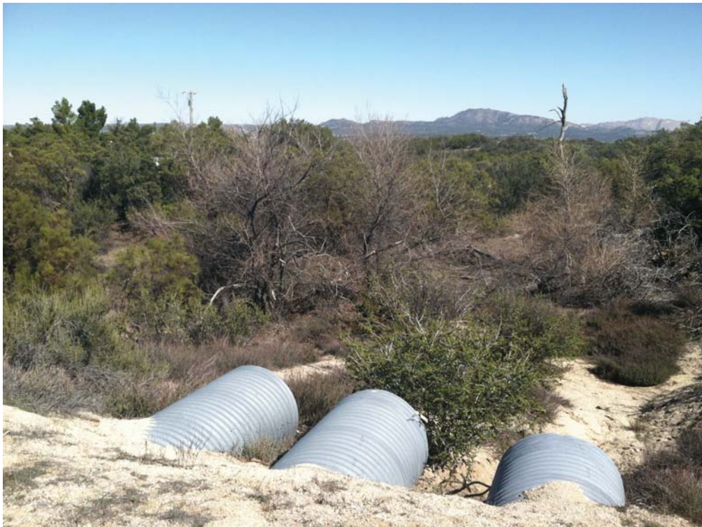
Photograph 6: Feature F Facing generally east. Photograph taken from existing access road.
