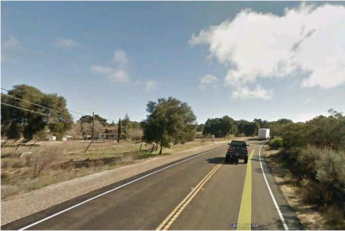
G. SR-94 looking northeast - Project route partially screened by intervening topography and vegetation.
