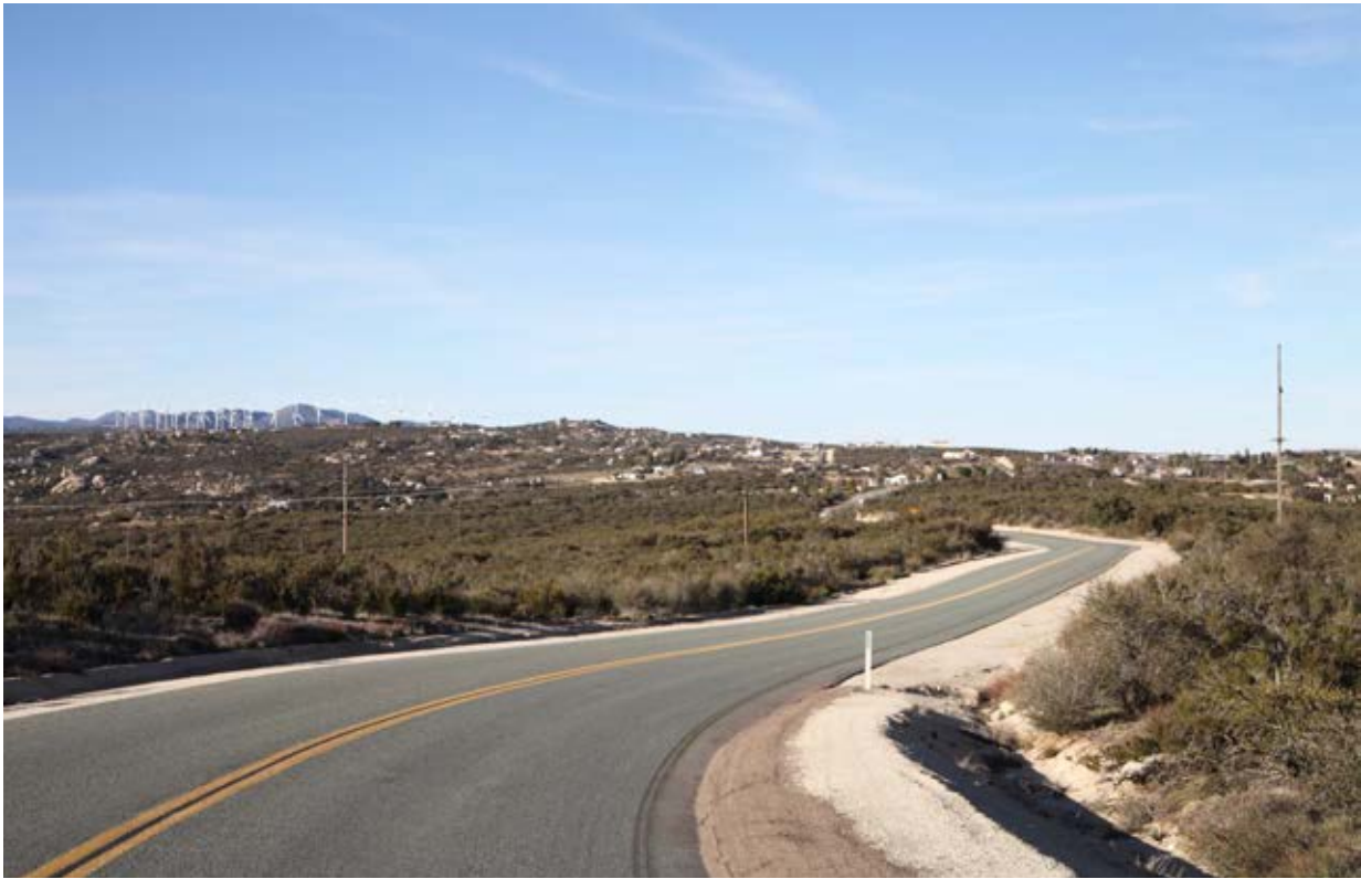
5. Tierra Del Sol Road looking north - Lower portions of existing poles screened by vegetation.
