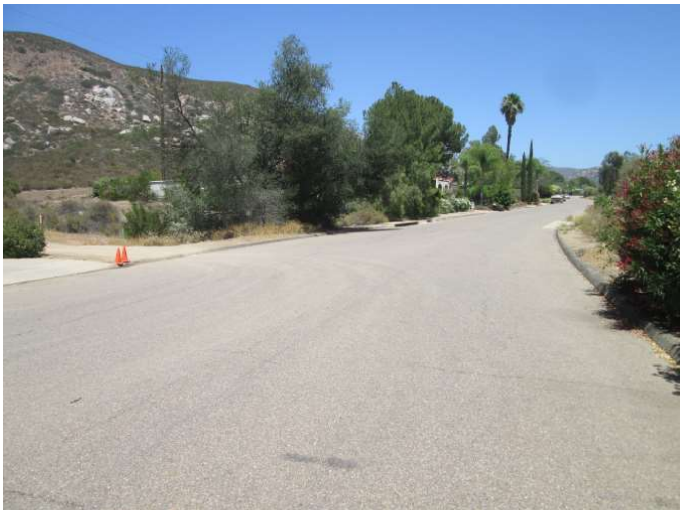
Photo 6: Access roads intersecting with paved community access roads were observed to be free of sediment track- out.
