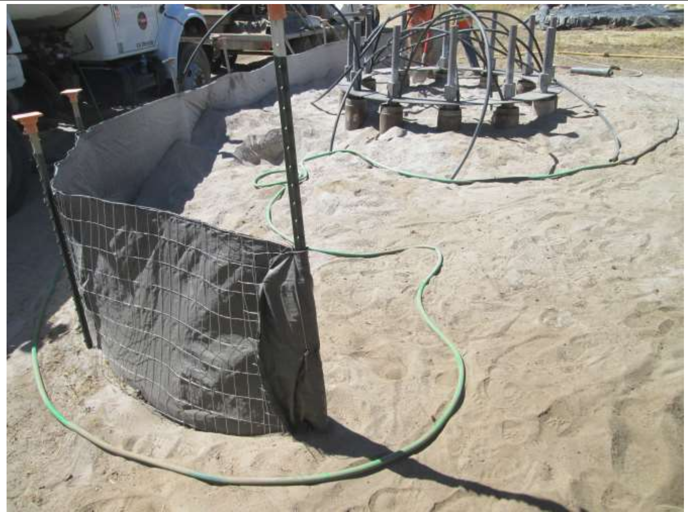
Photo 2: During grouting activities at micropile pole locations, silt fencing was observed utilized and intact/containing sediment in accordance with the project SWPPP.
