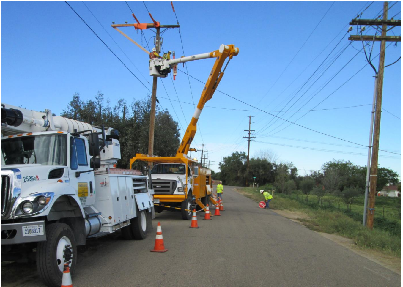
Photo 3: Traffic Control along Creelman Lane was observed being implemented in accordance with MM TRA-1 during pole topping/ wire spreading activities.
