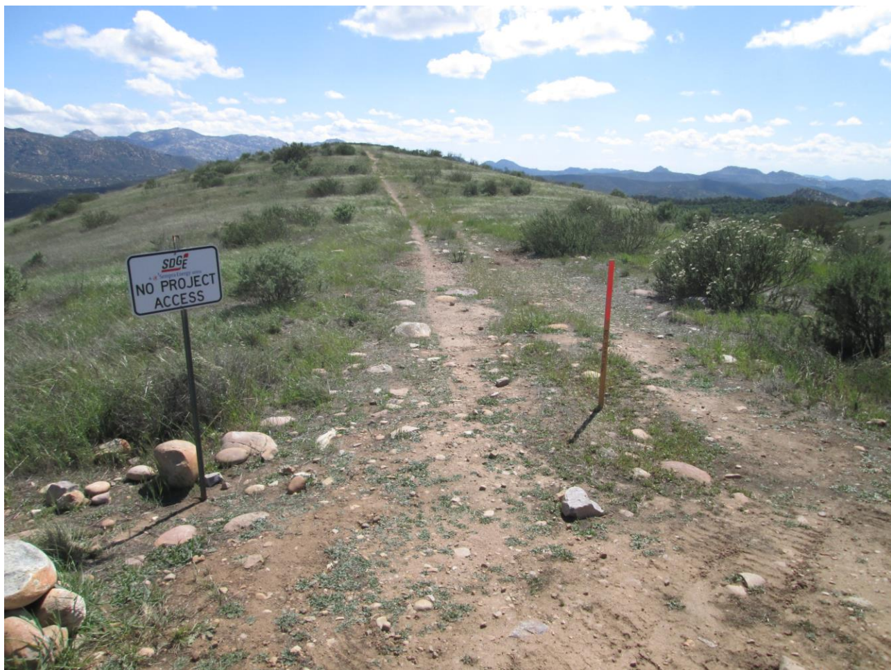
Photo 8: In order to facilitate awareness of approved access roads, signage and red-colored posts were placed in areas that could be mistaken for project roads indicating “NO PROJECT ACCESS.”
