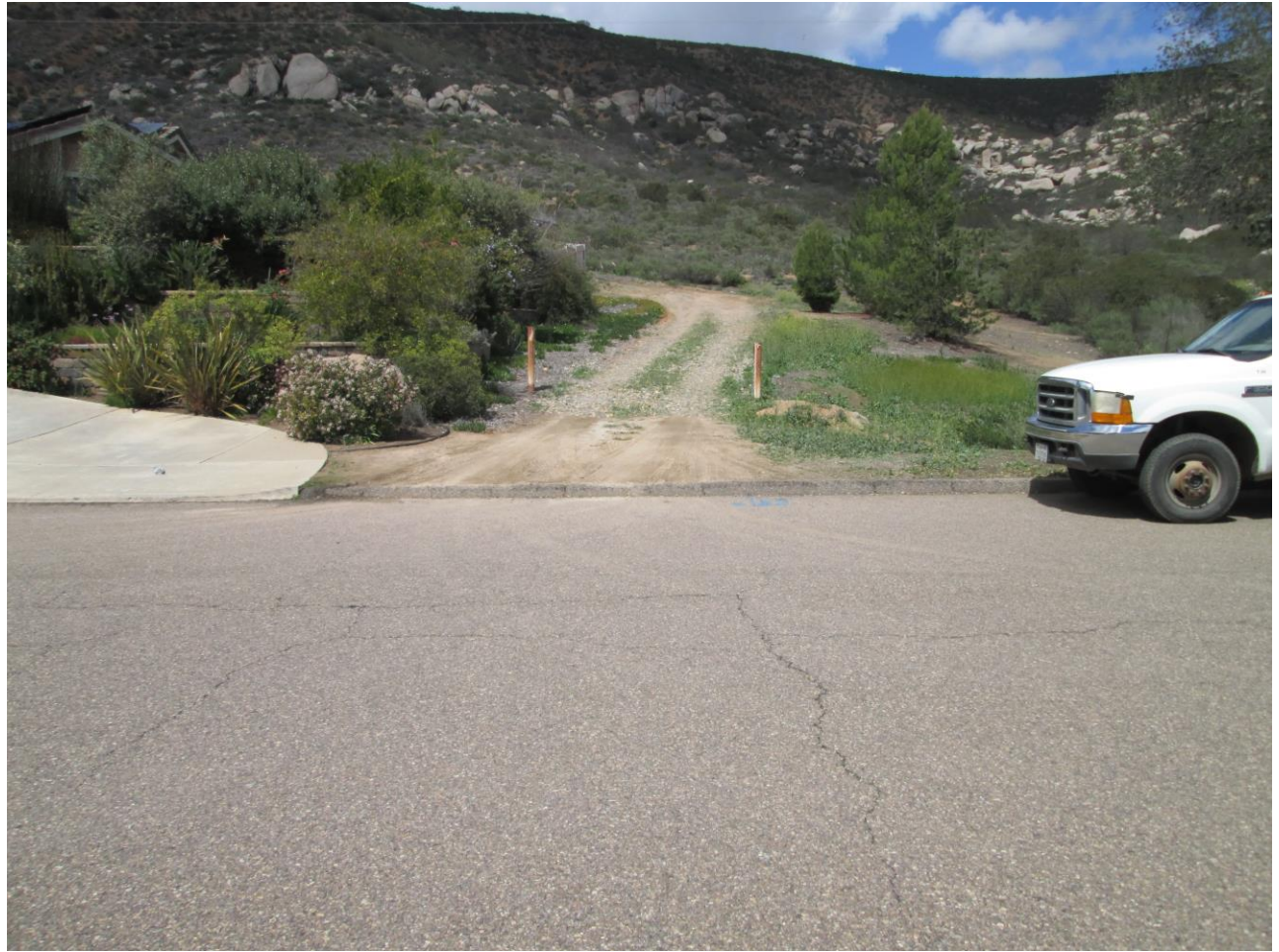
Photo 7: Points of ingress and egress to project pole locations were observed free of track-out in accordance with the Project SWPPP.
