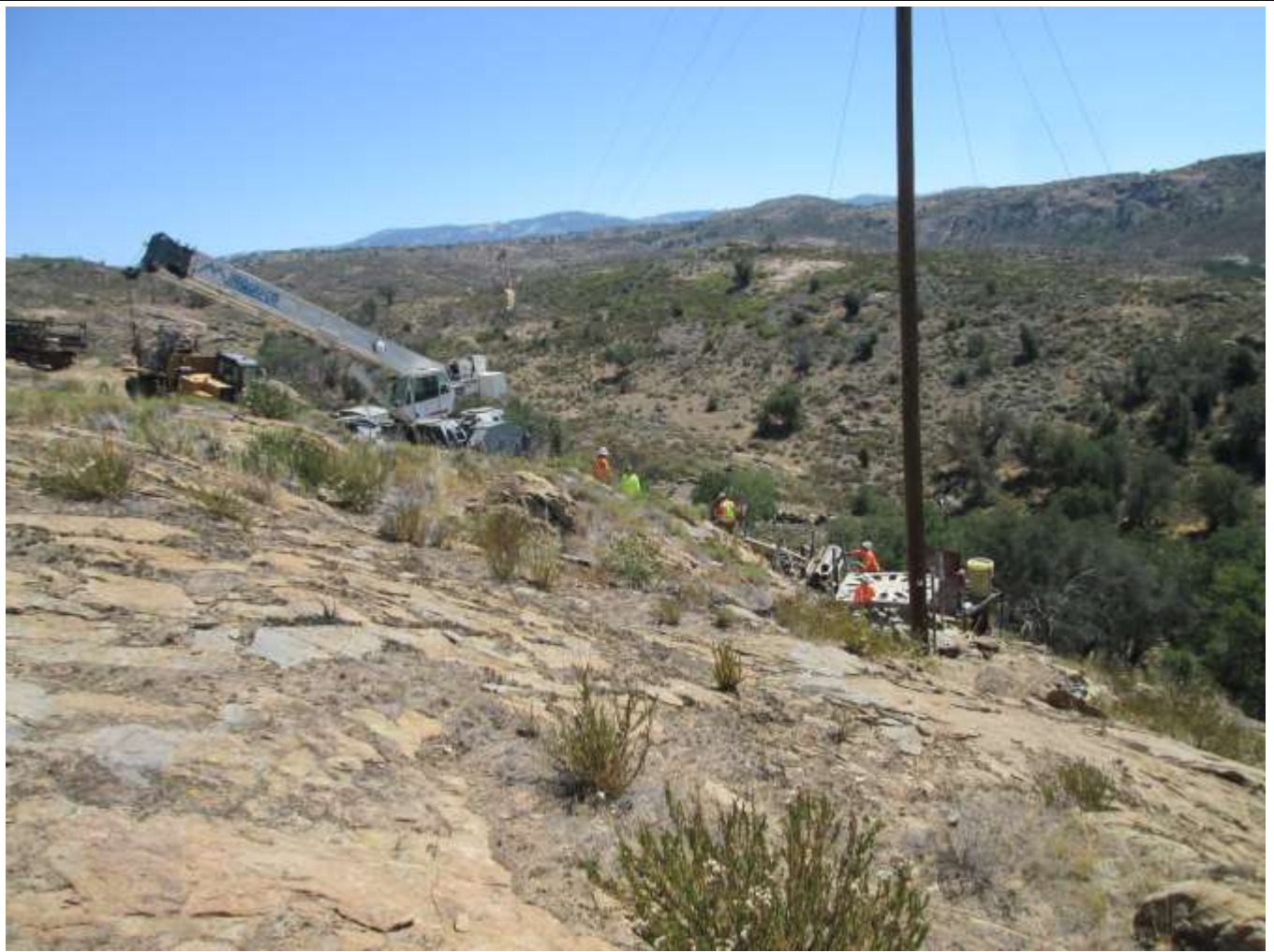
Photo 2: Crews were observed setting up micropile foundation staging equipment.
