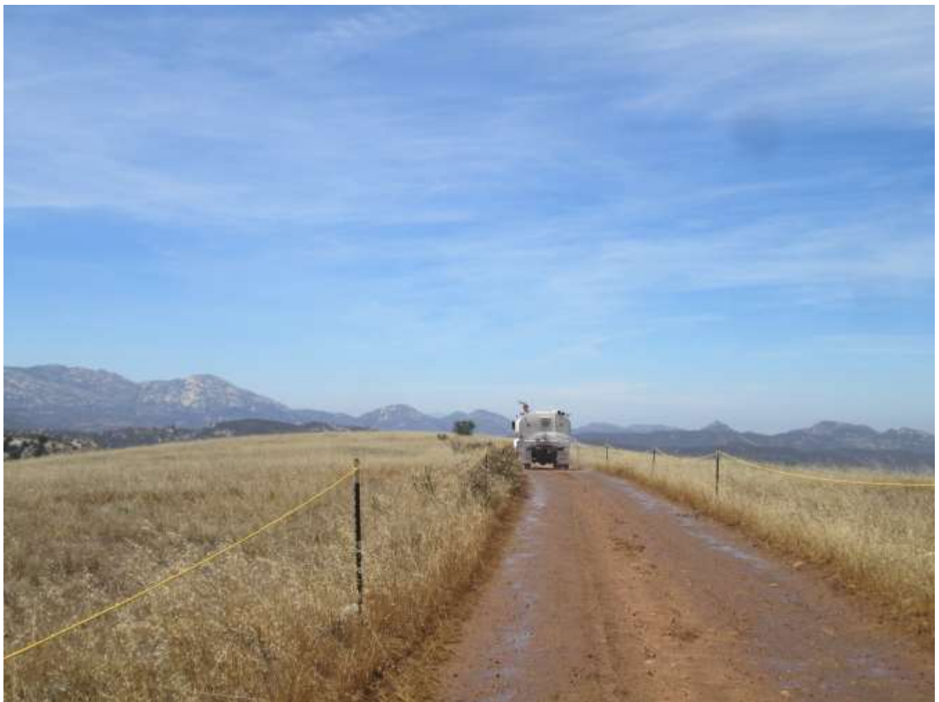
Photo 5: Water trucks were observed watering roads in order to ensure dust control in accordance with APM BIO-1.
