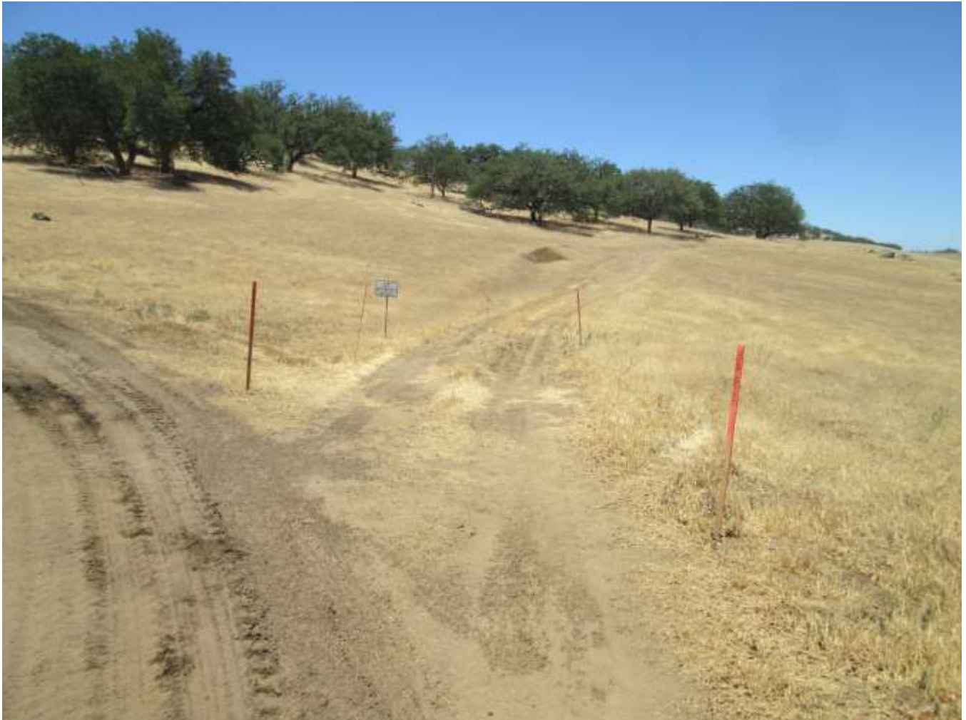
Photo 8: Orange-marked stakes were observed showing limits for approved turnaround areas and “No SDG&E Access” signs were installed to ensure that crews did not use the area behind the turnaround as an access road.
