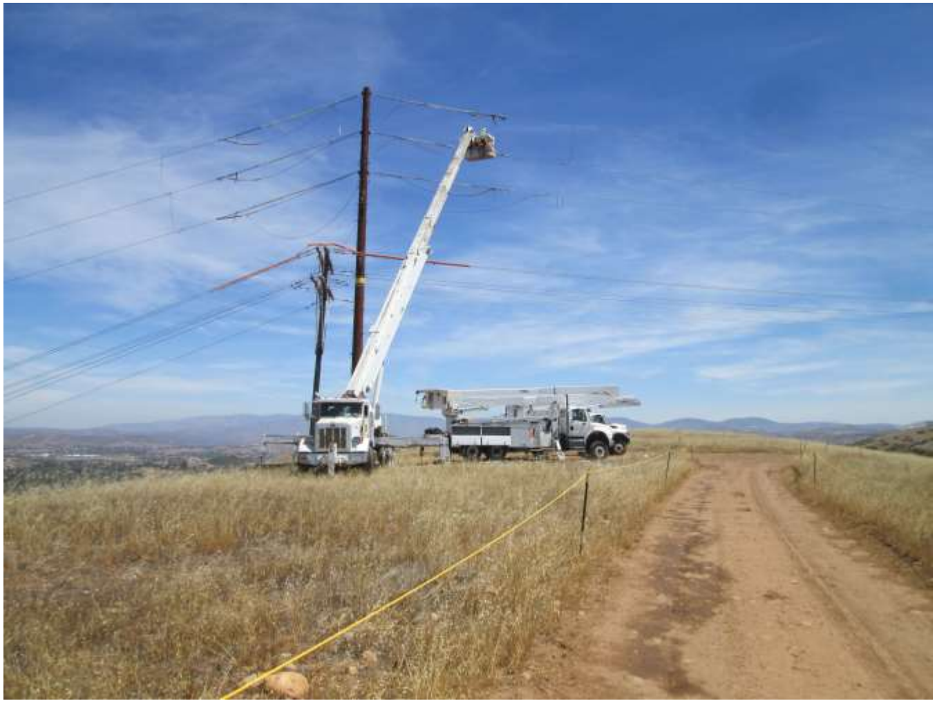
Photo 1: Construction crews were observed conducting wire stringing activities, which included dead-ending and sagging the wire (pictured above).
