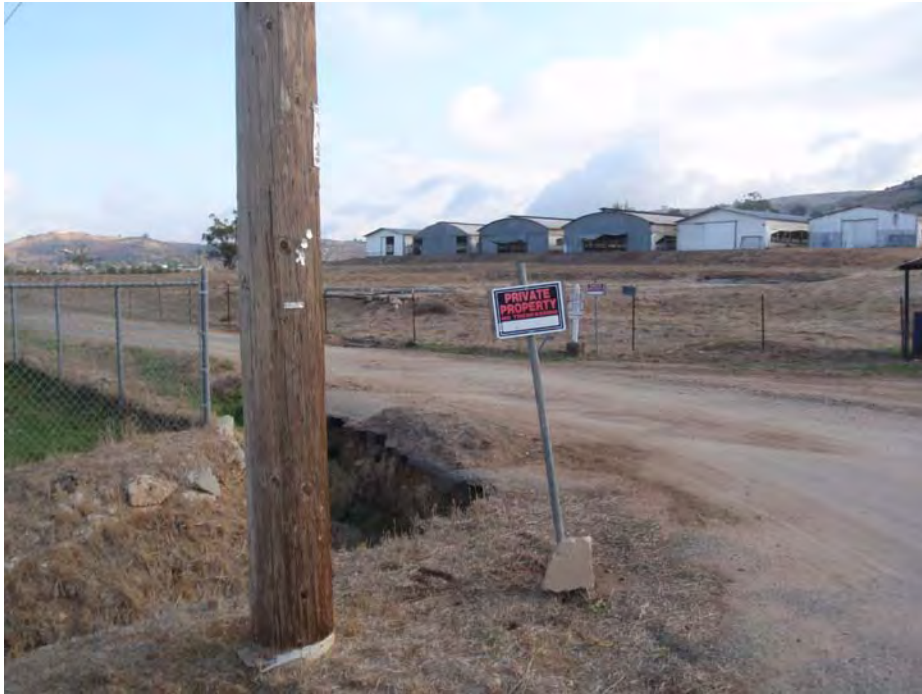
Pole R171. Photo taken looking east along the north side of Creelman Rd. Existing pole located at the top of a drainage feature. Removal: access pole from road and pull out with boom truck and wench to minimize impacts. Will require BMPs to avoid impacts to drainage. Location #14
