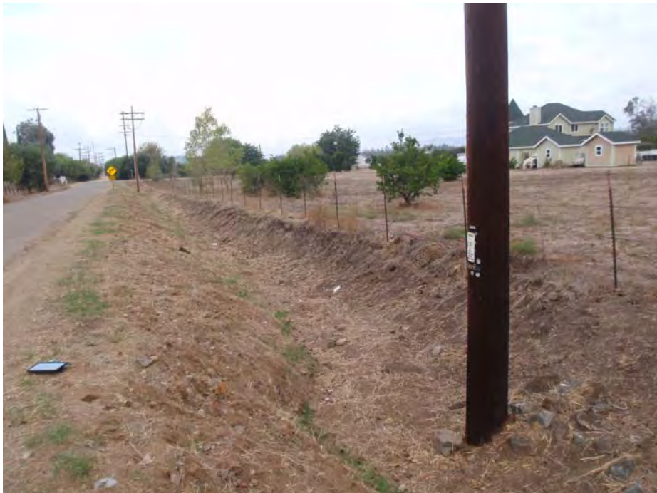
Pole R11, pole removal. Photo taken looking west along Creelman Rd. Pole is located within a drainage feature. Options for removal are cut at base and leave, or access pole from road and pull out with boom truck and wench to minimize impacts. Location #16
