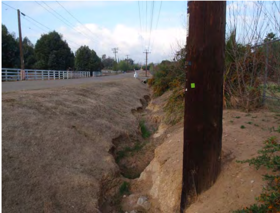
Pole R13. Photo taken looking west along Creelman Rd. Existing pole located a drainage feature. Removal: access pole from road and pull out with boom truck and wench to minimize impacts. May require back hoe to dig out from exposed bedrock. Location #17
