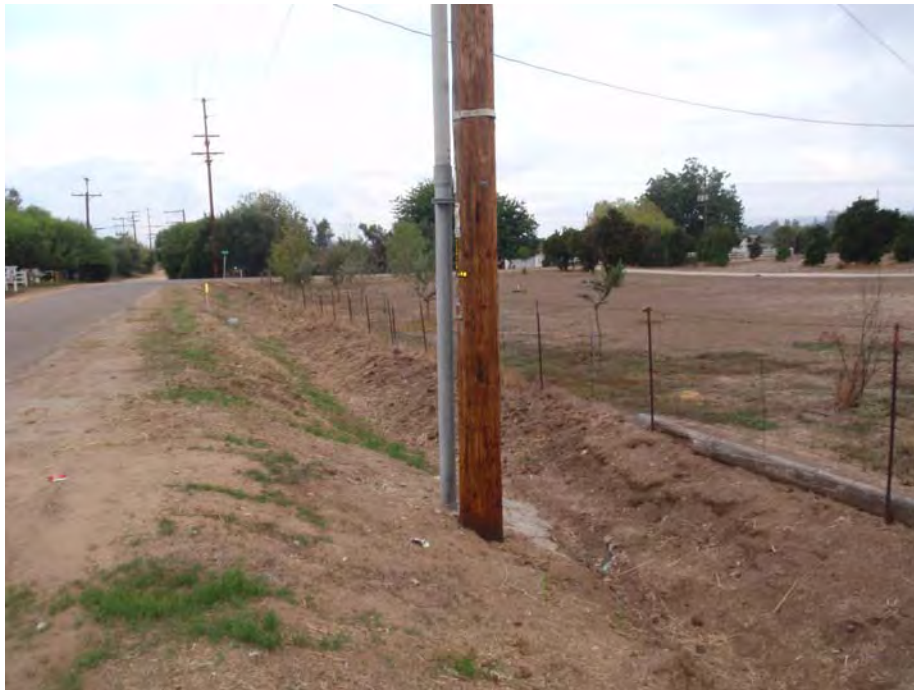
Pole R10, pole removal. Photo taken looking west along Creelman Rd. Pole is located within a drainage feature. Options for removal are cut at base and leave, or access pole from road and pull out with boom truck and wench to minimize impacts. Location #12
