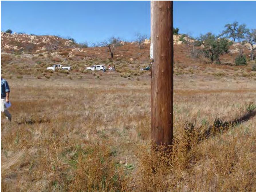
Pole P104. Photo taken looking northwest towards access road. The pole will be relocated to this side of the access road, outside of the wetland area. Removal of pole will temporarily disturb the wetland area, but will minimize disturbance during maintenance activities of pole (access to pole).
