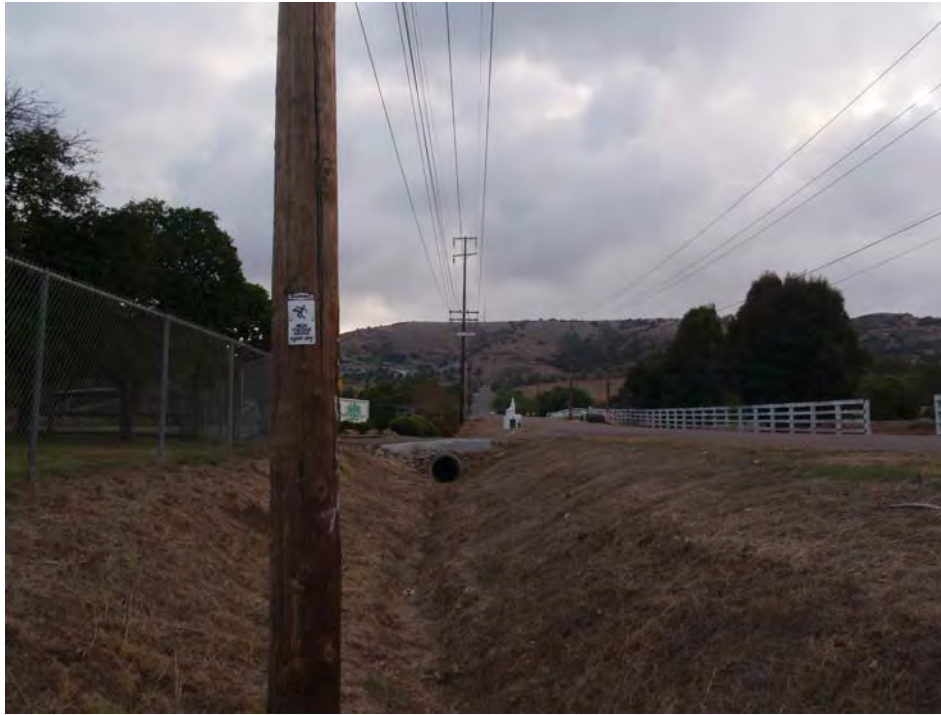
Pole R169. Photo taken looking east along Creelman Rd. Existing pole located a drainage feature. Removal: access pole from road and pull out with boom truck and wench to minimize impacts. Loc#13
