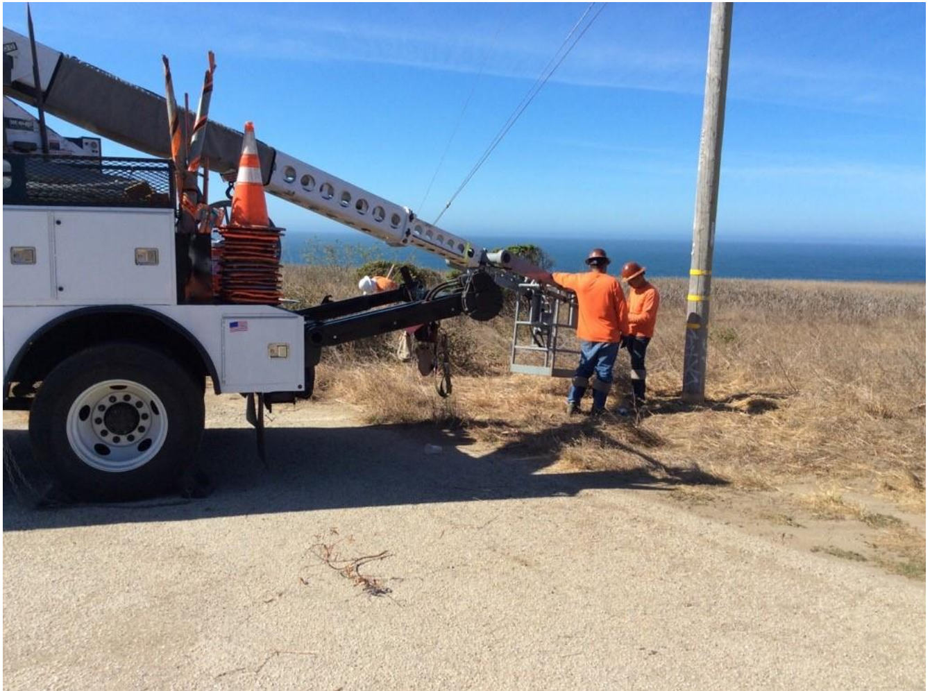
Photo 2: Crew installing pole guy wire anchors.
