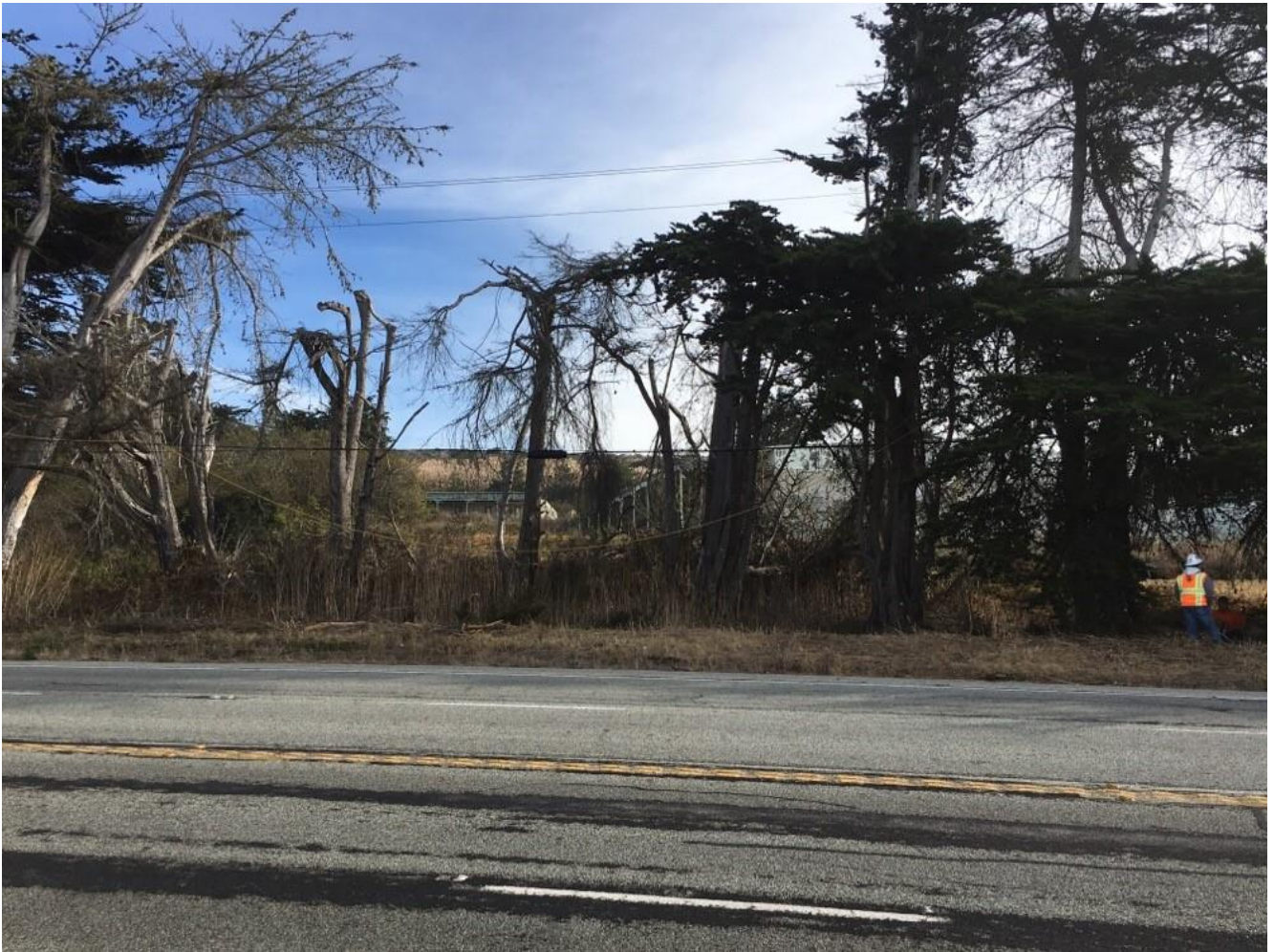
Photo 4: Aerial line installation.
