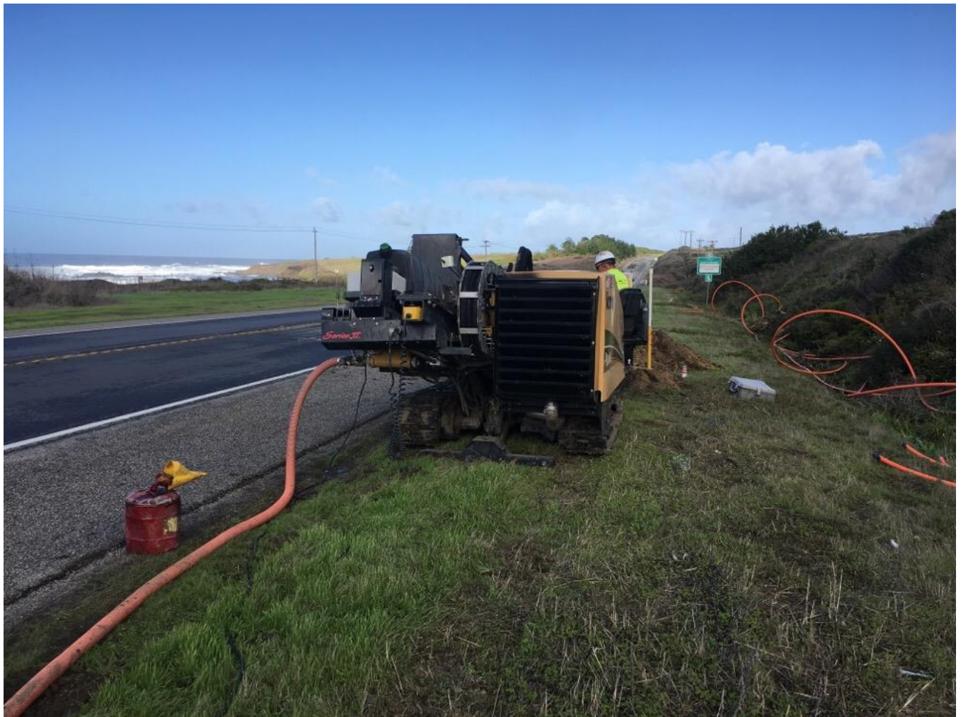
Photo 2: HDD drill in operation.
