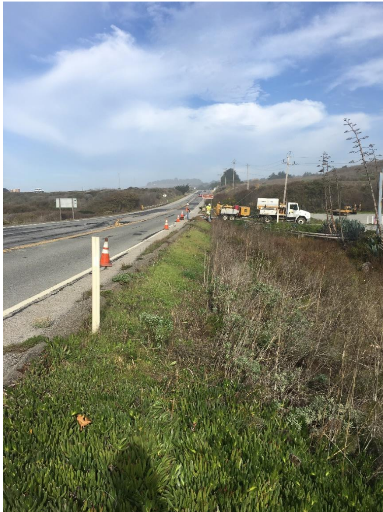
Photo 5: HDD installation along Highway 1, near brewery.
