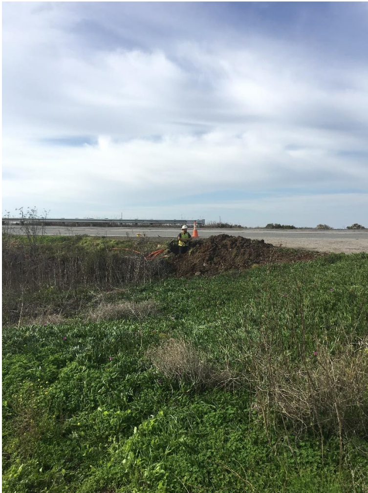
Photo 4: HDD installation along Highway 1 near brewery.
