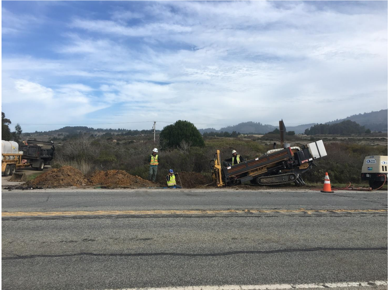
Photo 6: HDD crew retrieving stuck HDD drill head.
