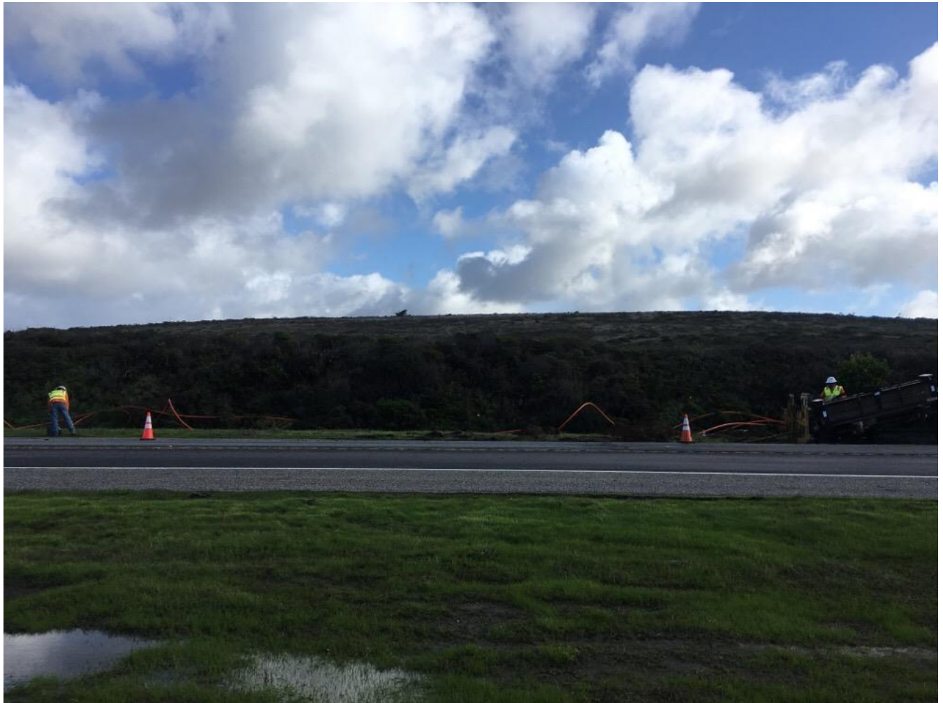
Photo 1: HDD installation across from Pigeon Point Road.
