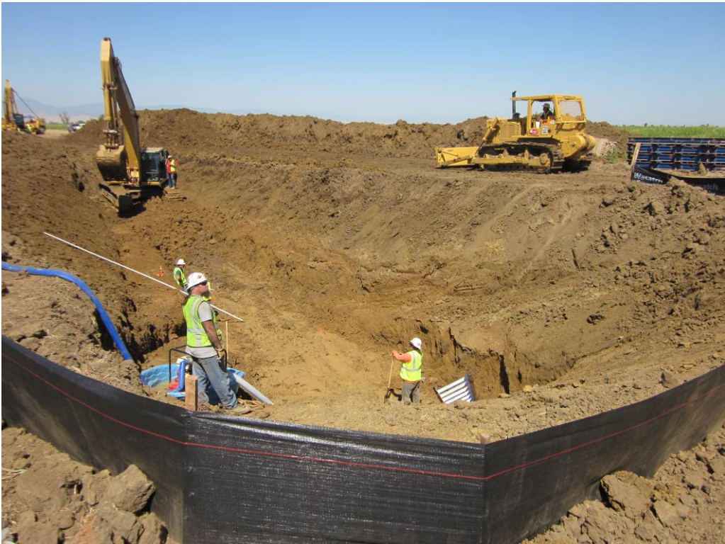
Photo 4: Auger bore hole excavation at D-31. Hole includes the creation of wildlife escape ramps on both sides. Silt fence has been installed between hole and D-31.
