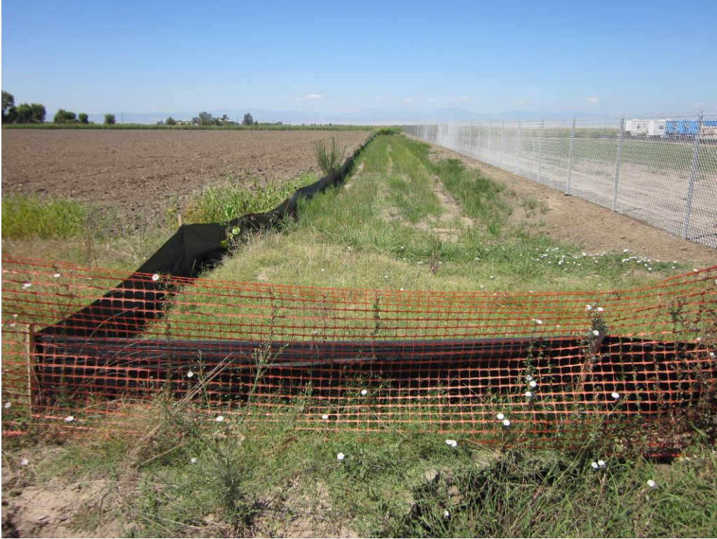
Photo 3: Sensitive resource exclusion fencing along the southern edge of the remote well pad site.
