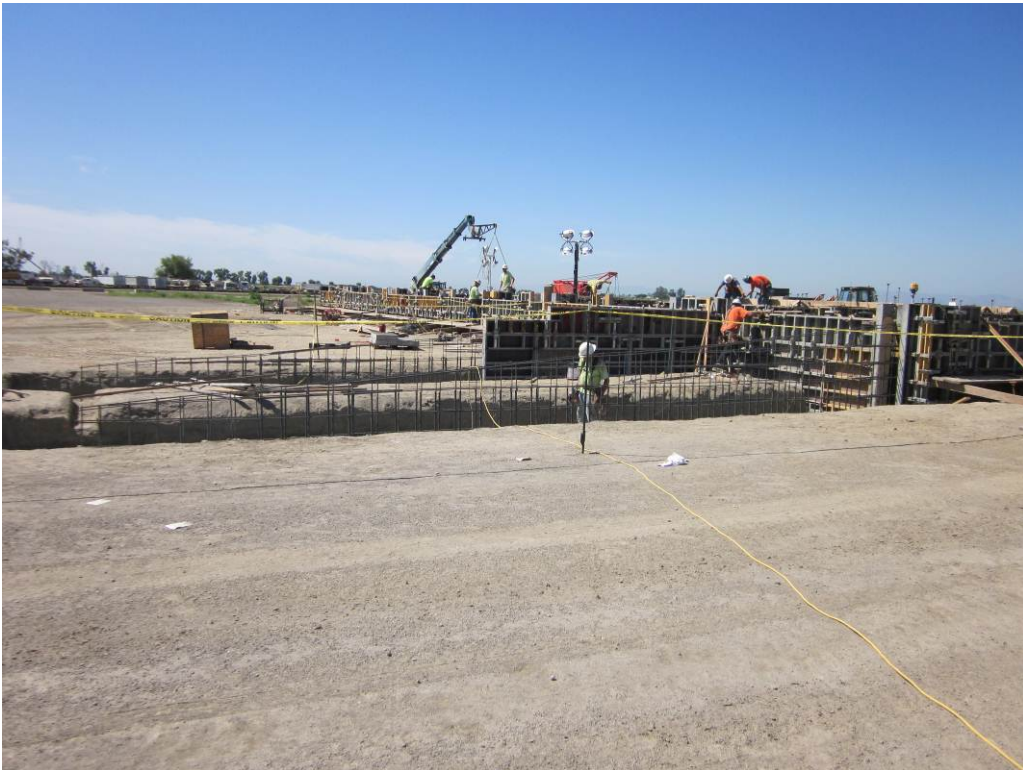
Photo 2: Foundation work at the compressor station site.
