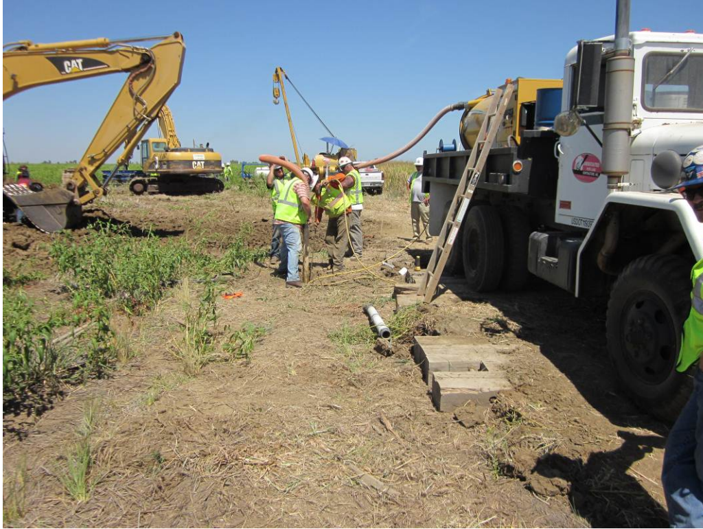
Photo 5: Potholing along the natural gas connecting pipeline alignment (at D-31).
