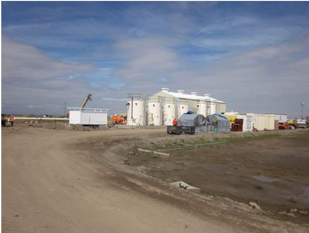
Photo 1: Saltwater storage tank at the Remote Well Pad site being prepared for painting. The containment dike around the tank has also been completed.
