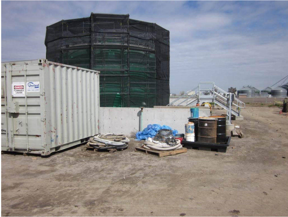
Photo 1: Saltwater storage tank at the Remote Well Pad site being prepared for painting. The containment dike around the tank has also been completed.
