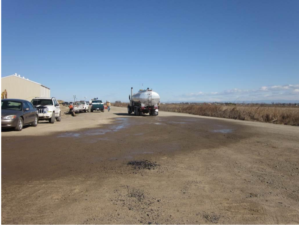
Photo 3: Water truck being utilized to control dust emissions from the Compressor Station site and along McAusland Road.
