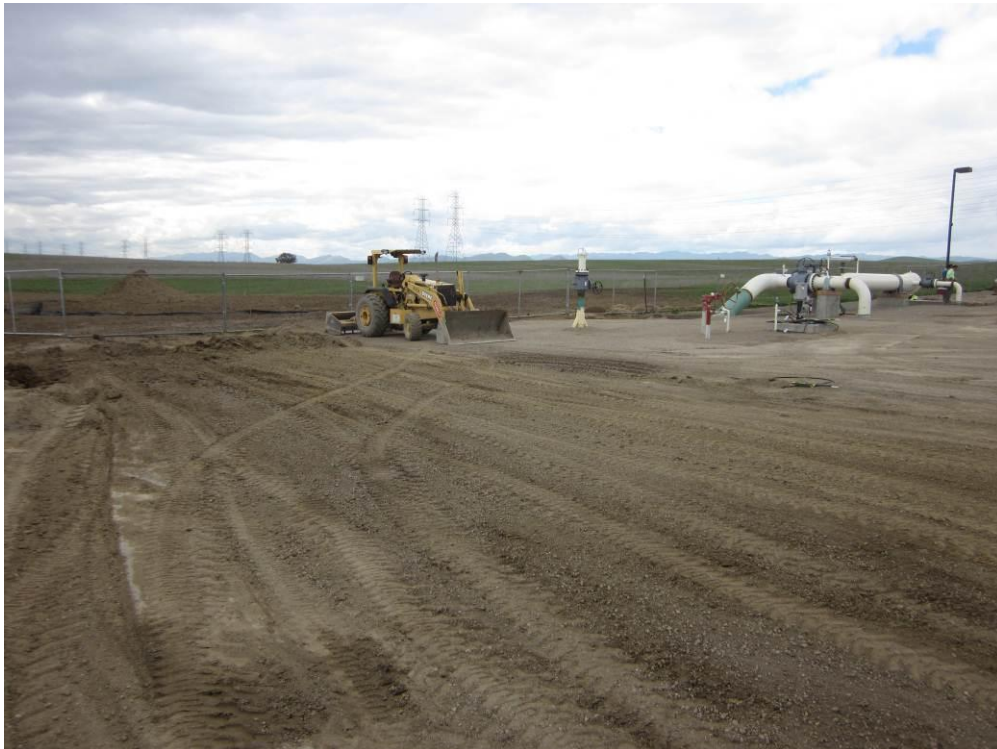
Photo 6: Backfilling and final grading at the Metering Station site was underway.
