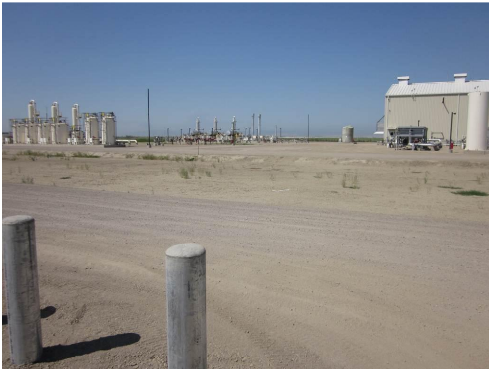
Photo 4: The Compressor Station site has been graded and road base installed.
