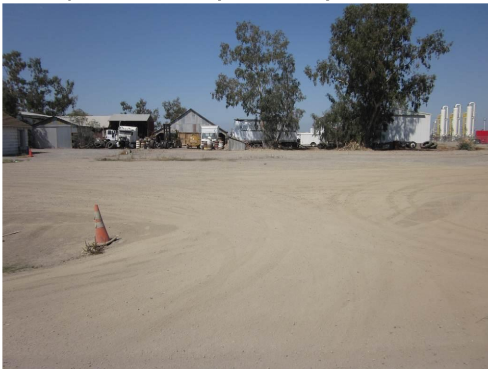
Photo 2: Temporary office trailers and silt fence have been removed from the area immediately south of the Compressor Station site.
