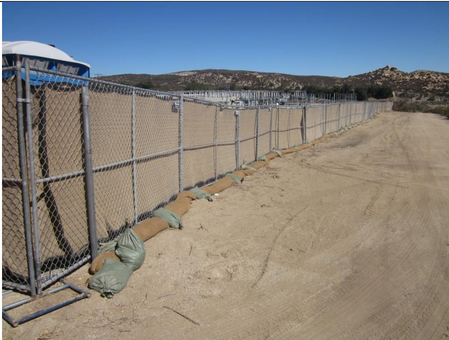
Photo 6: Erosion control measures consisting of straw wattles were observed installed and being maintained in accordance with MM-HYD-1. Visual screening fencing was in good condition in accordance with MM-VIS-3e.
