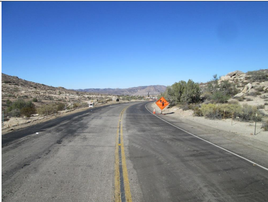
Photo 2: Signage is placed along Old Highway 80 notifying motorists of construction activities in accordance with MM-TRA-1.
