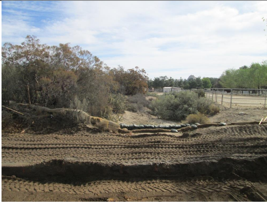
Photo 1: Erosion control devices were observed being maintained in accordance with MM-HYD-1.
