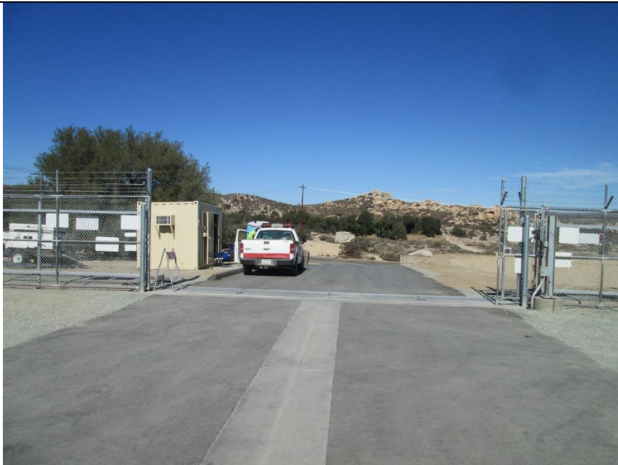
Photo 6: Fire patrols were observed to be present during construction activities at the Boulevard Substation Rebuild in accordance with MM-FF-1.
