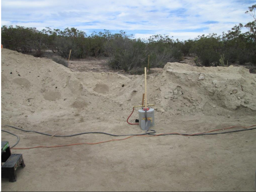
Photo 3: Fire equipment was observed being maintained in areas of active construction in accordance with MM-FF-1.
