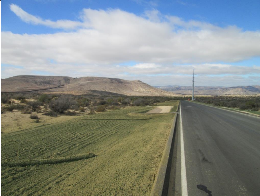
Photo 5: Restoration efforts associated with temporary work spaces adjacent to the ECO substation access road continued during this reporting period. Hydroseed has been placed on restoration areas in accordance with MM-BIO-1D.
