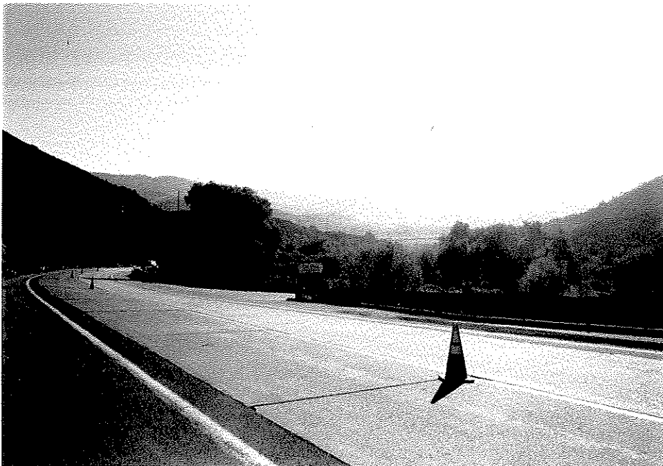
US80-8- North of Pine Valley (in distance) – note large oak trees – looking south
