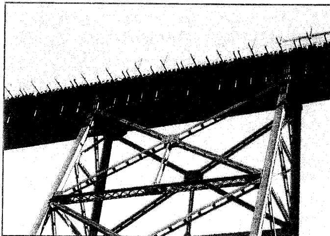
Upper portion of trestle looking east.
