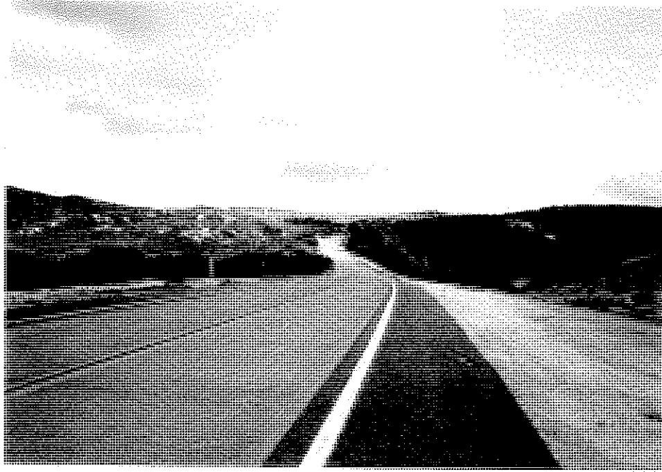
***US80-21- Between La Posta and Miller Valley Rd.- dip and curve in road, looking south
