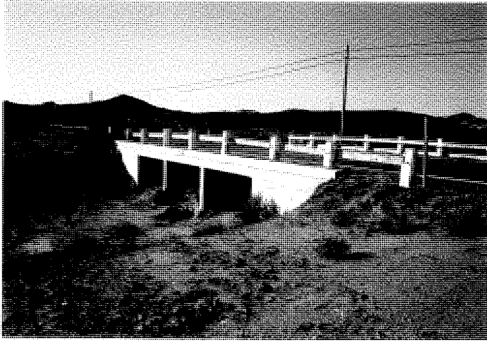
US80-37- Bridge #57C-229, at Horse Creek, looking northwest
