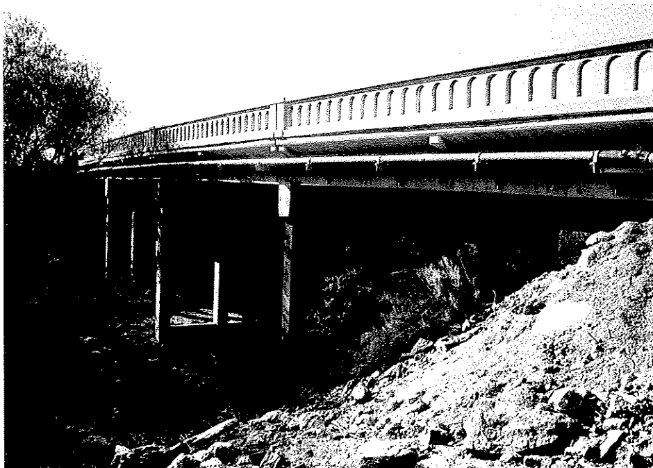
US80-34- Bridge #57C-227, five pile concrete bents
