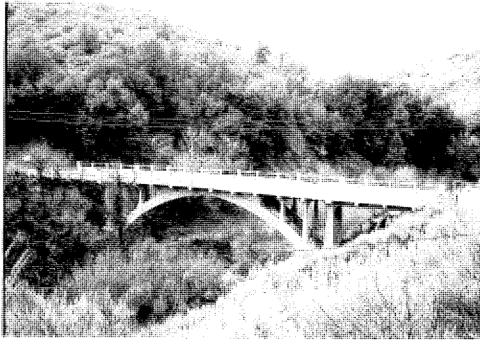
US80-11- Old bridge on Pine Valley Creek – abandoned – just west of Bridge #57C-335
