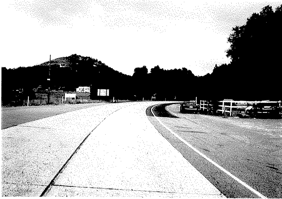
US80-3- At Riverside Rd. – looking east, PCC surface and curve in road
