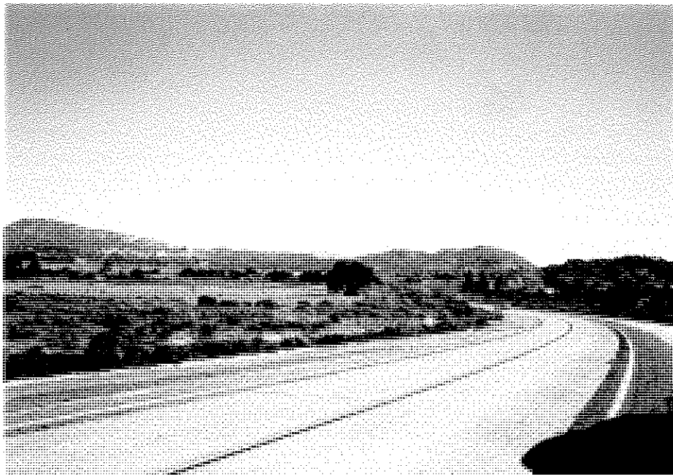
***US80-27- Just south of Boulevard, looking south
