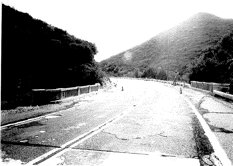
US80-16- Bridge #57C-338, at Cottonwood Creek, looking south
