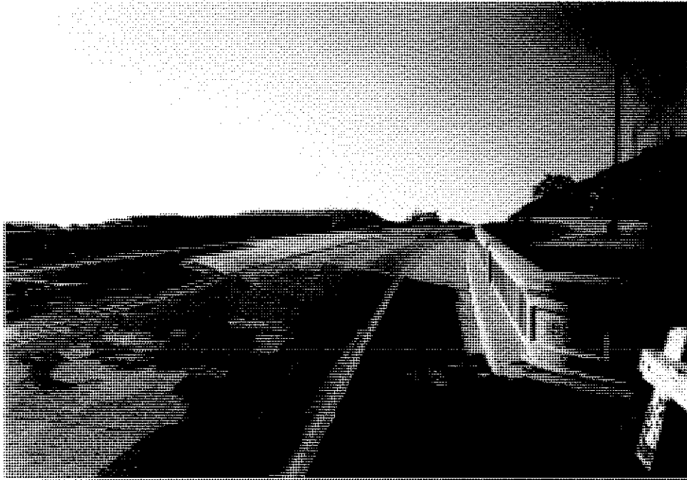
US80-29 Bridge #57C-226, Jacumba Overhead, looking southeast
