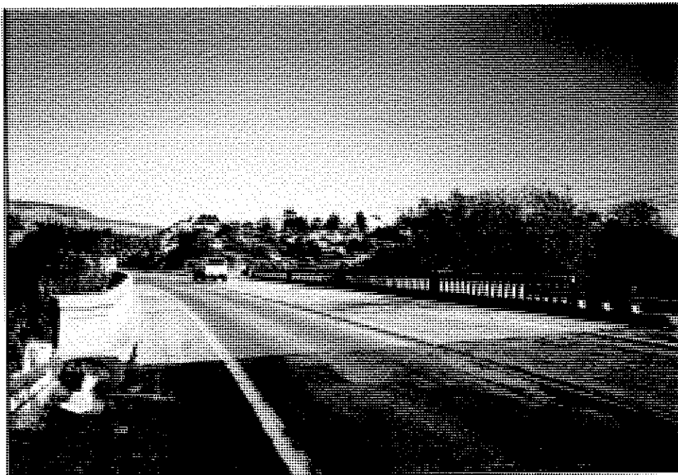
US80-33- Bridge #57C-227, over Boundary Creek, looking east
