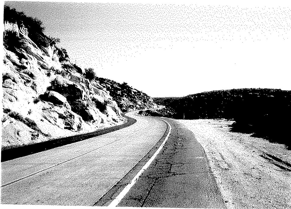
***US80-22- Between La Posta and Miller Valley Rd., "S" curve, looking south
