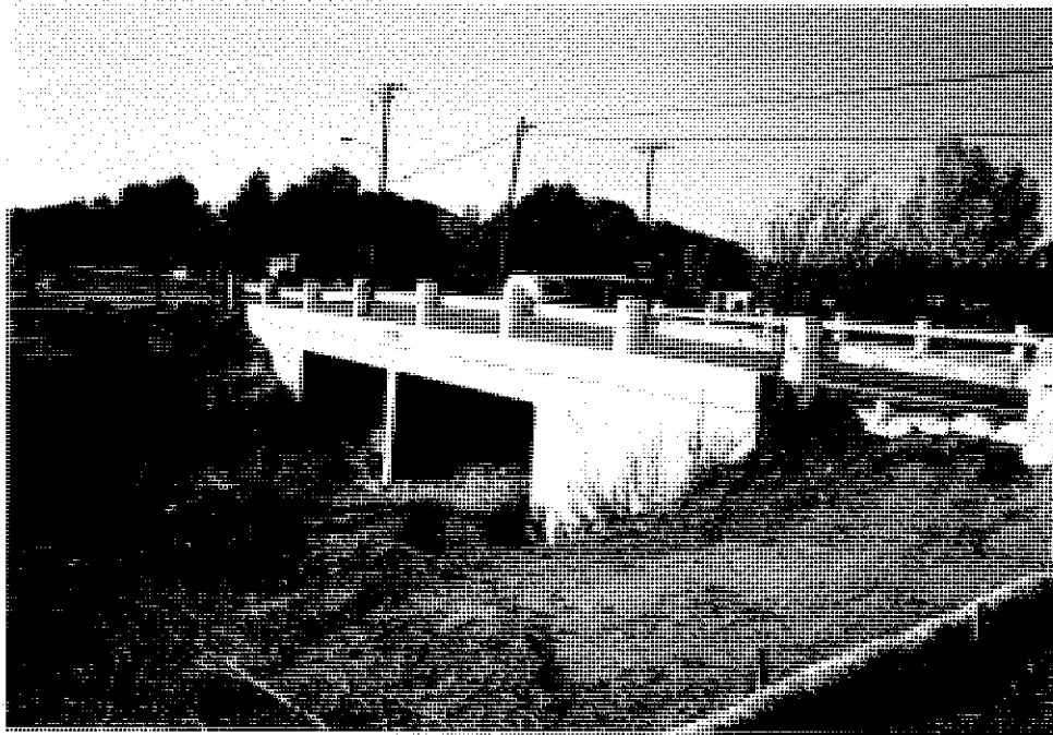
US80-36- Bridge #57C-228, at Meadow Creek, looking northwest
