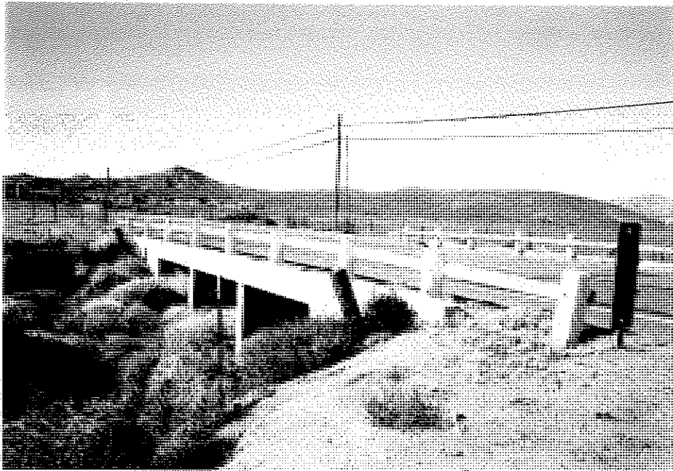
US80-38- Bridge #57C-230, at Flat Creek, looking west
