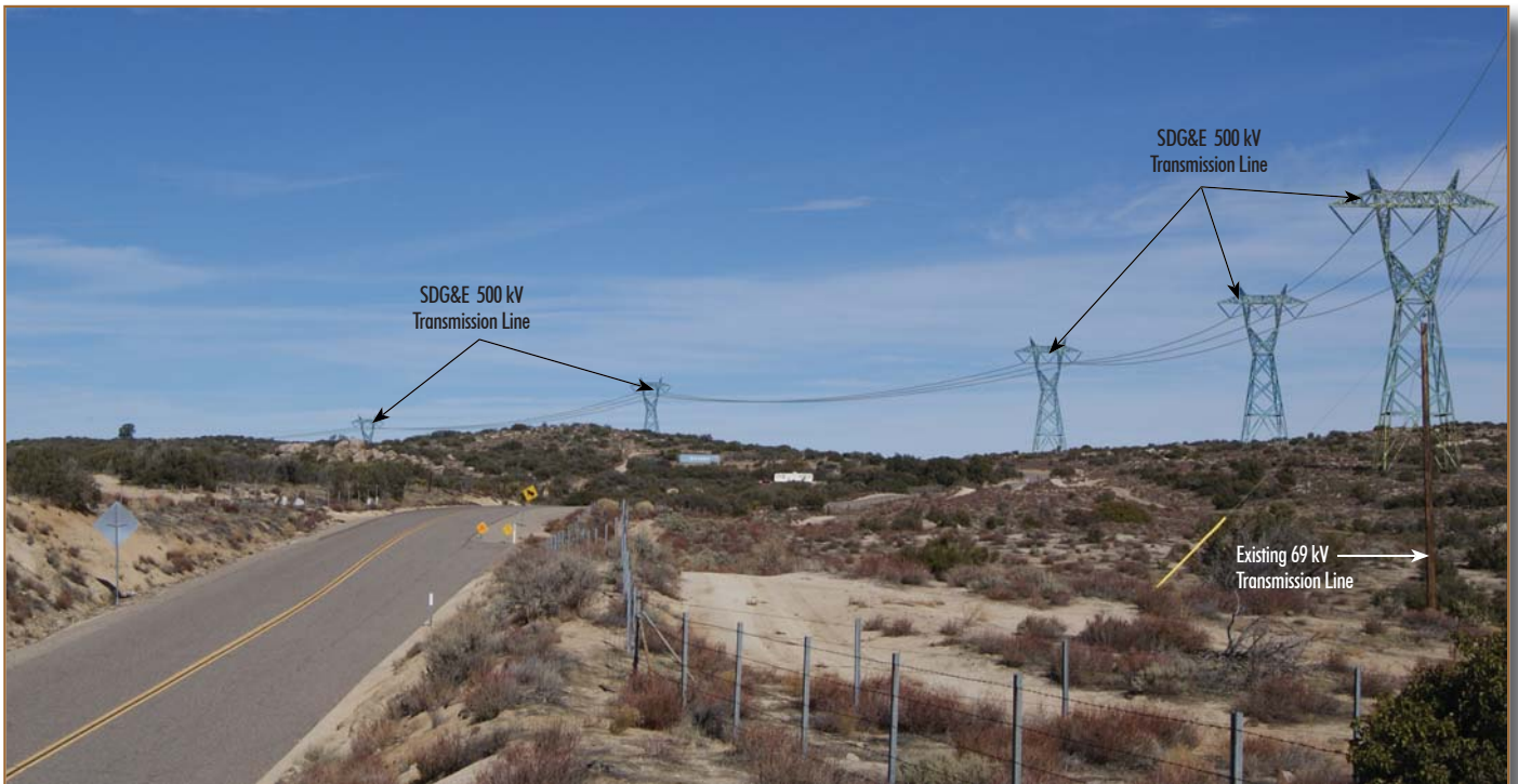
SDG&E Sunrise Powerlink – 500 kV transmission line (Approved)
