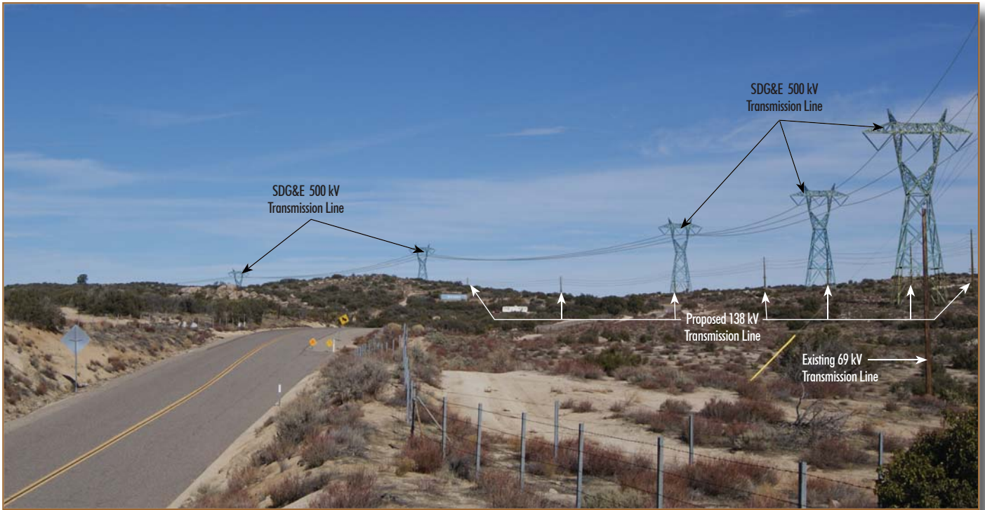
SDG&E Sunrise Powerlink – 500 kV transmission line (Approved) and Tule Wind Project – 138 kV transmission line
