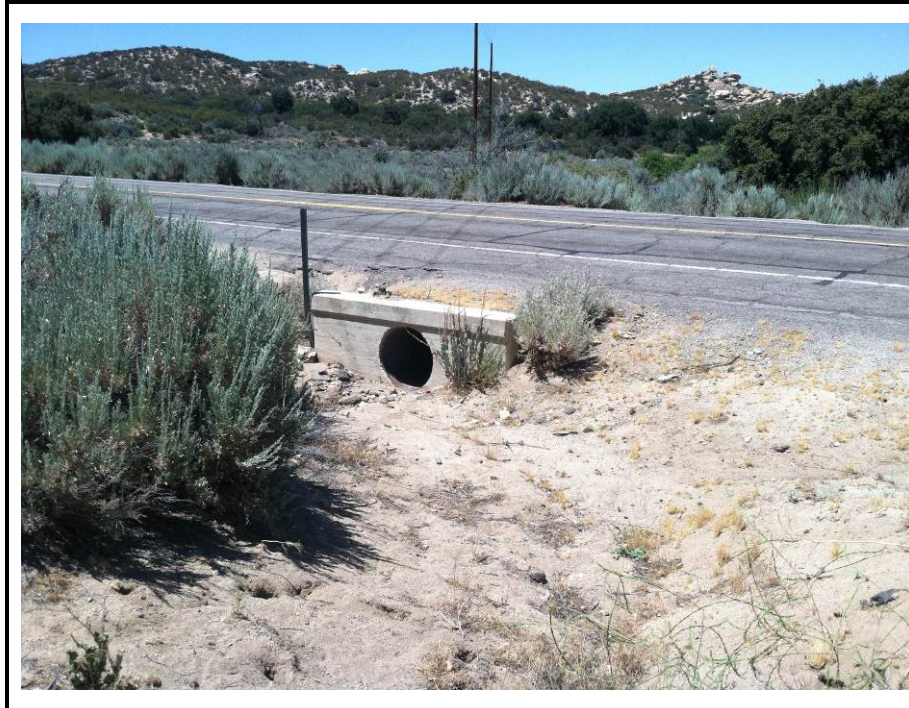
Photograph 3: View of the southern side of the culvert replacement facing north.
