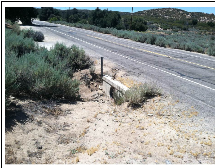
Photograph 4: View of the southern side of the culvert replacement facing west.
