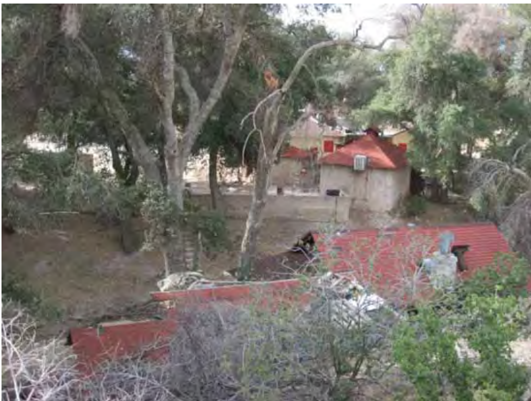
Figure 4.16 Overview of the historic component at TuleEP-08.
