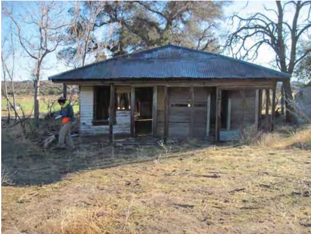
Figure 4.14 Overview of Tule-CW-25.
