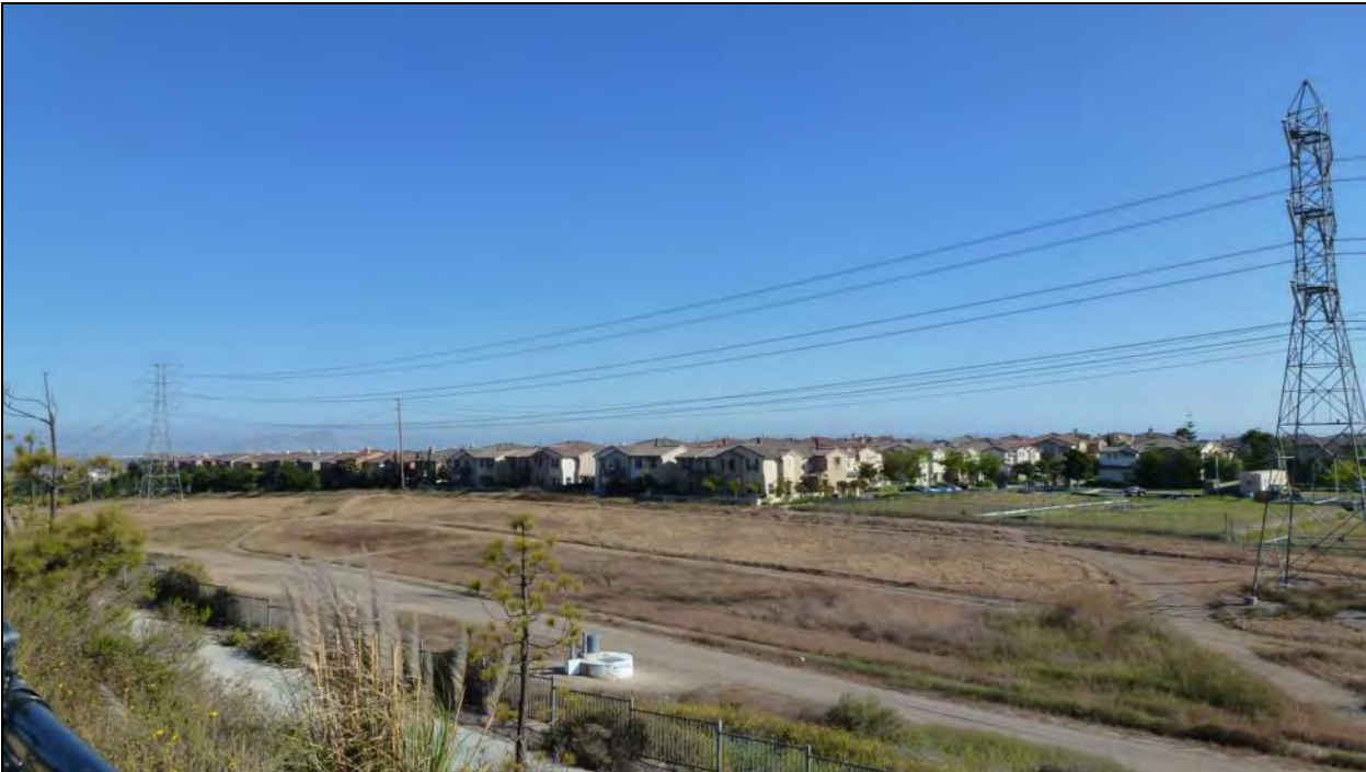
Figure 4.1-8: Existing Foreground Views
