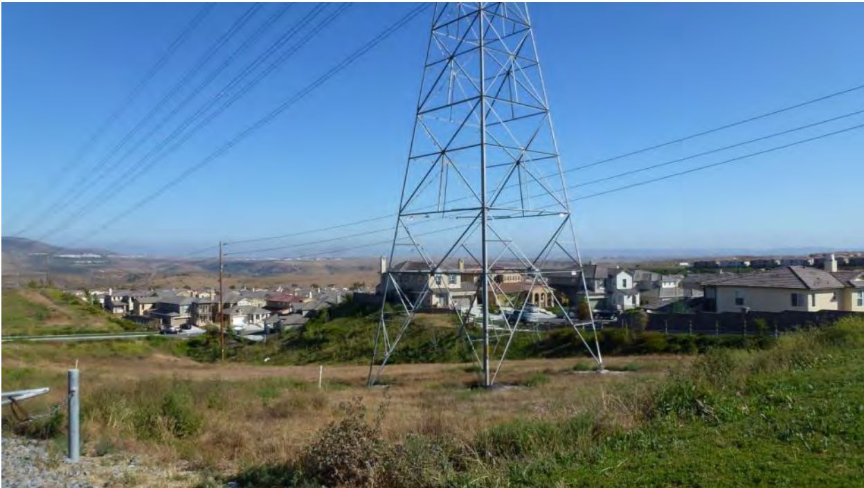
Figure 4.1-11: View South along the Transmission Corridor
