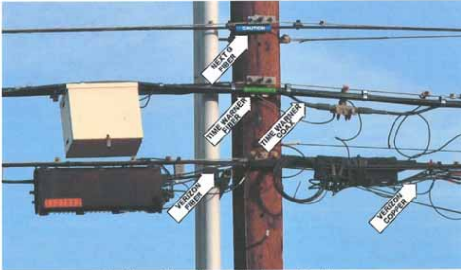
Time Warner: Fiber cable overlashed to coaxial cable Verizon: Fiber cable overlashed to twisted pair copper cable LOCATION: Springdale Street near Dorita Drive (indicated by hexagon on map)
