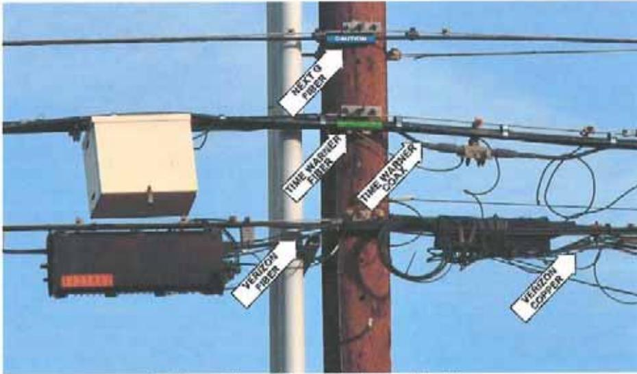
Time Warner: Fiber cable overlashed to coaxial cable
