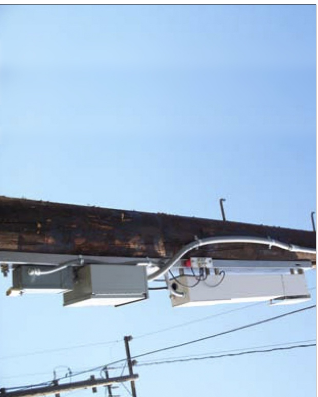
Photo 6: Ground Buss Connections
