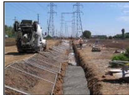
Underground duct bank construction
