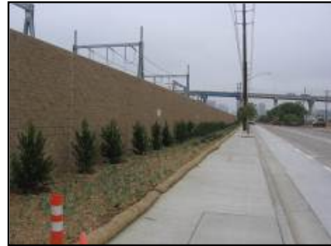
A typical 10-foot-tall Concrete Masonry Wall
