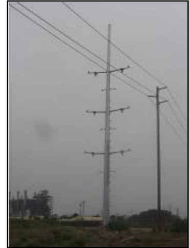
Existing OMPL steel cable pole riser to be removed
