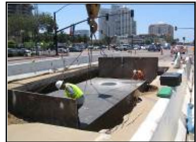
Precast vault placement via use of a crane
