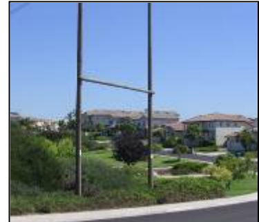
A typical temporary guard structure
