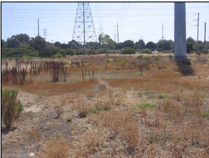
Photo 3: View of 230 kV Tangent Pole Structure Looking East
