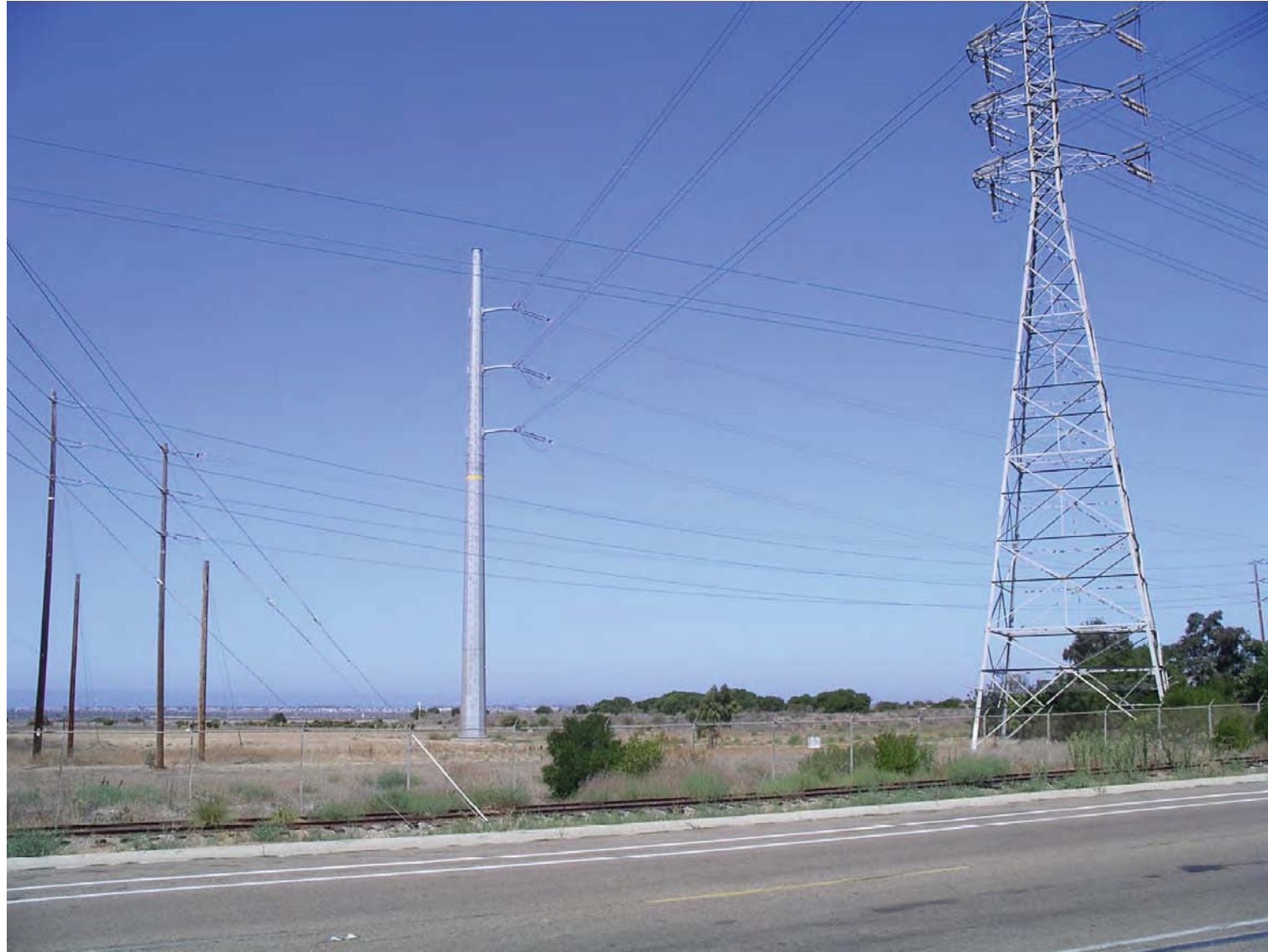
Existing Condition (View from Bay Boulevard, looking west)
