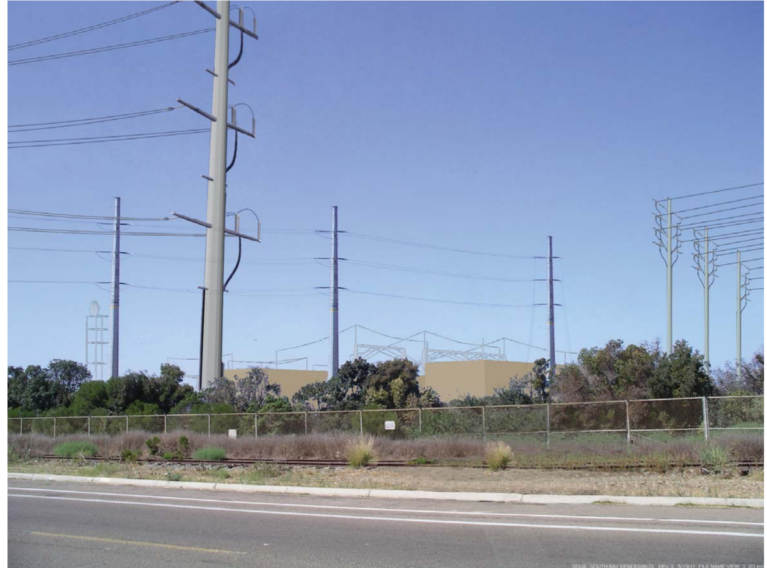
Visual Simulation of the air-insulated substation at the proposed Bay Boulevard Substation site (View from Bay Boulevard north of Palomar Street, looking southwest)
