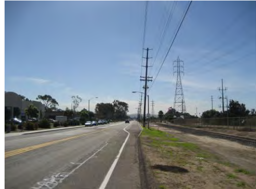
Photo 8: View south from Bay Boulevard south of the L Street exit toward transmission easement
