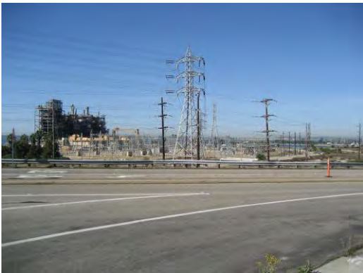
Photo 9: View west from L Street and Bay Boulevard intersection toward South Bay Substation
