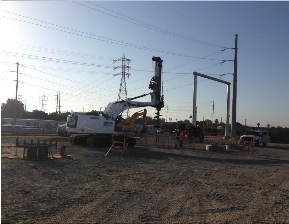
Photo 2: Drilling for tower foundations at the Bay Boulevard Substation 230kV pad.
