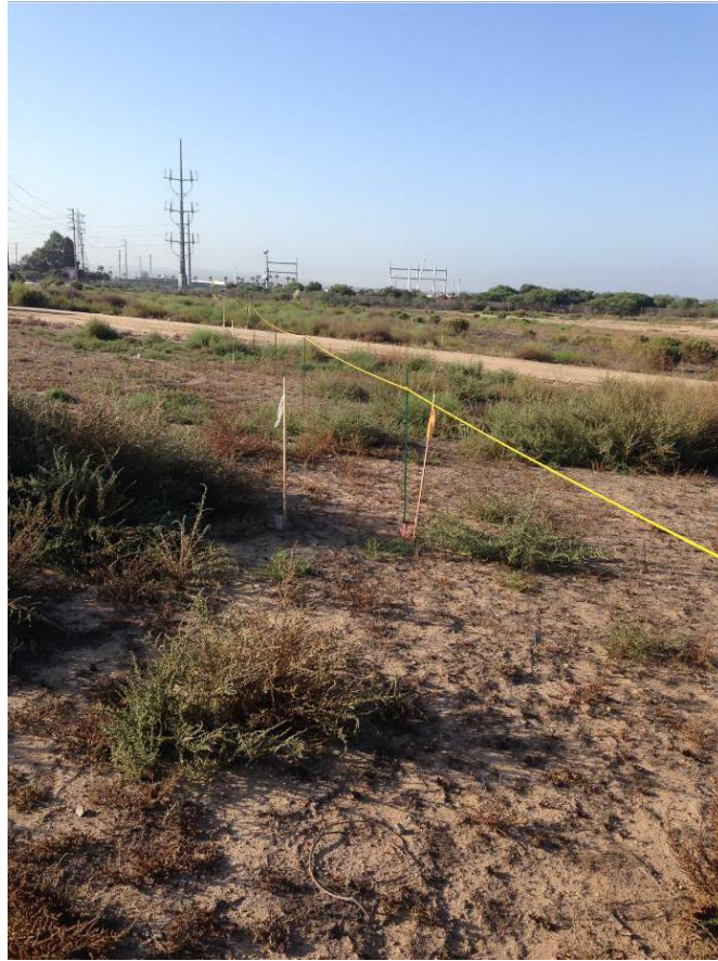
Photo 4: Prior work occurring along the transmission line alignment, work limits were delineated on the ground.
