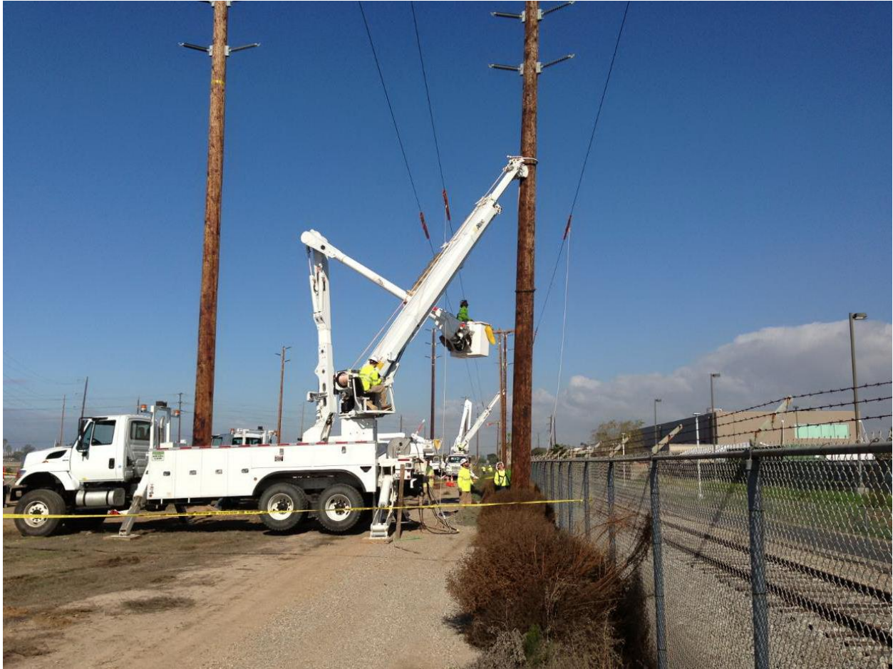
Photo 3: Crews were observed removing 69kV poles along the transmission line alignment.
