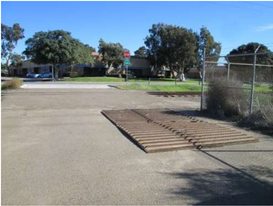
Photo 5: Rattle plates were observed stationed at the point of ingress/egress to the Bay Boulevard Substation location in order to minimize sediment track-out onto paved areas in accordance with MM HYRDO-1 and the project SWPPP (BMP-2-07, Tracking Controls).
