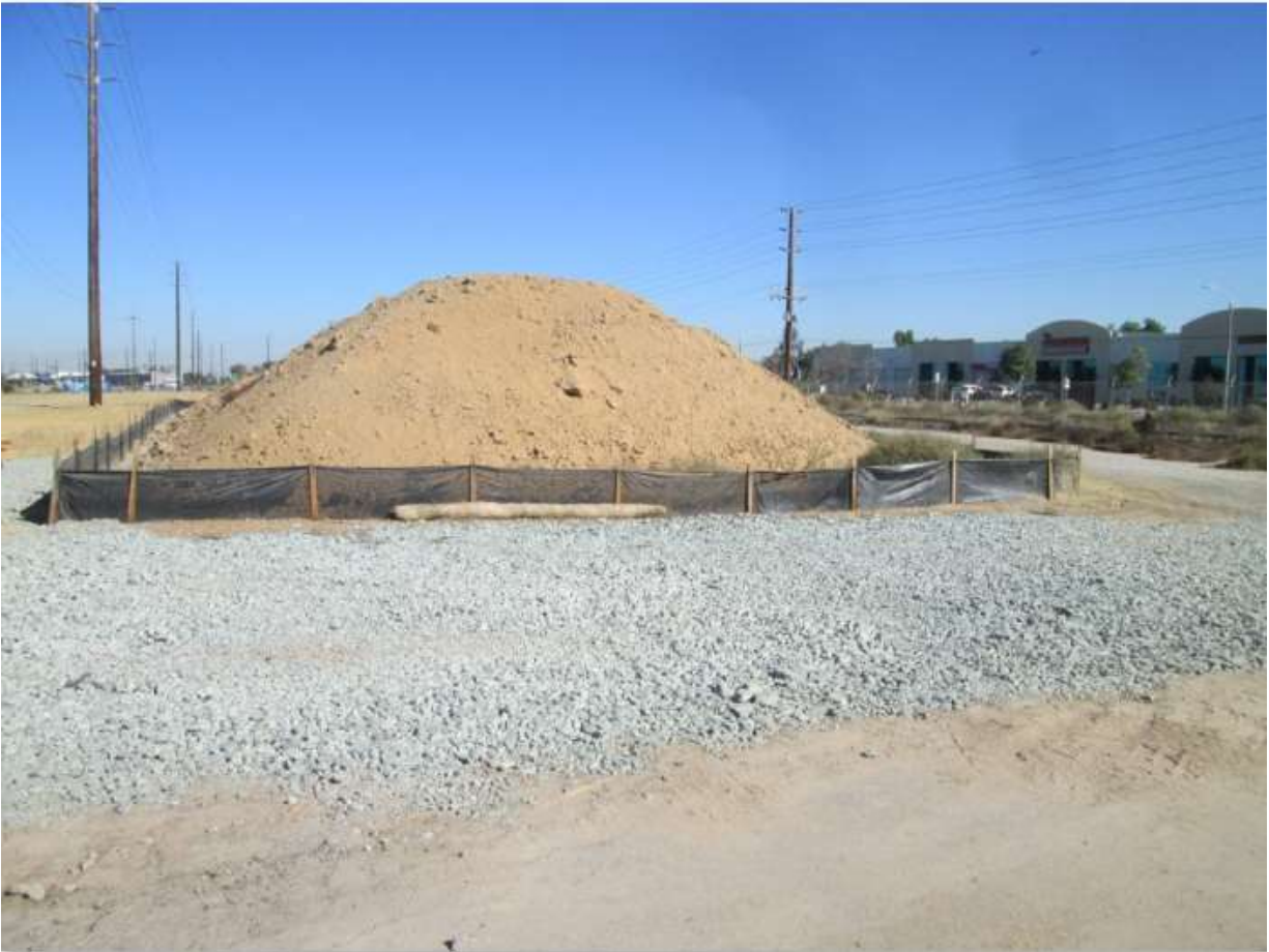
Photo 3: Sediment control BMPs, such as silt fencing around stockpiled topsoil, were being maintained in accordance with the project SWPPP (MM-HYDRO-01).
