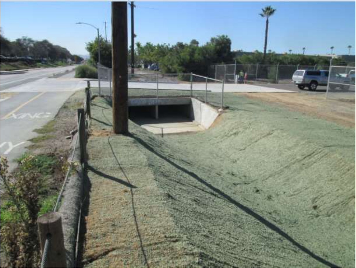
Photo 2: Hydromulch applied at the Bay Boulevard Substation entrance.
