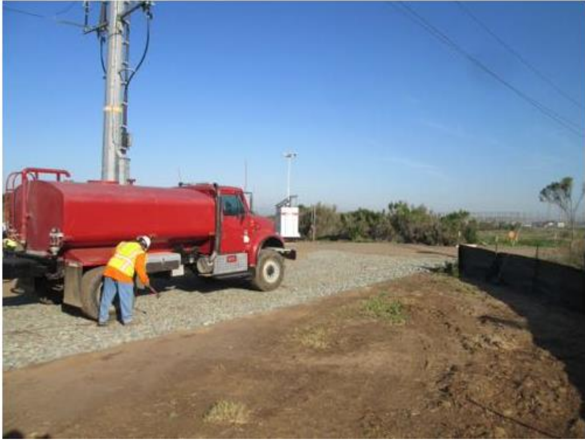
Photo 5: A water truck driver manually removing dirt/mud from the water truck tire tread before exiting the site to prevent sediment track-out in accordance with MM HYDRO-1 and MM BIO-5.
