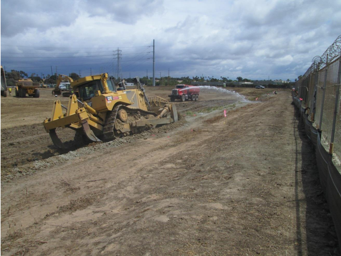
Photo 3: Water trucks were observed being utilized to water grading areas in order to minimize dust emissions in accordance with APM AIR-01. Monitors were observed present during these activities.
