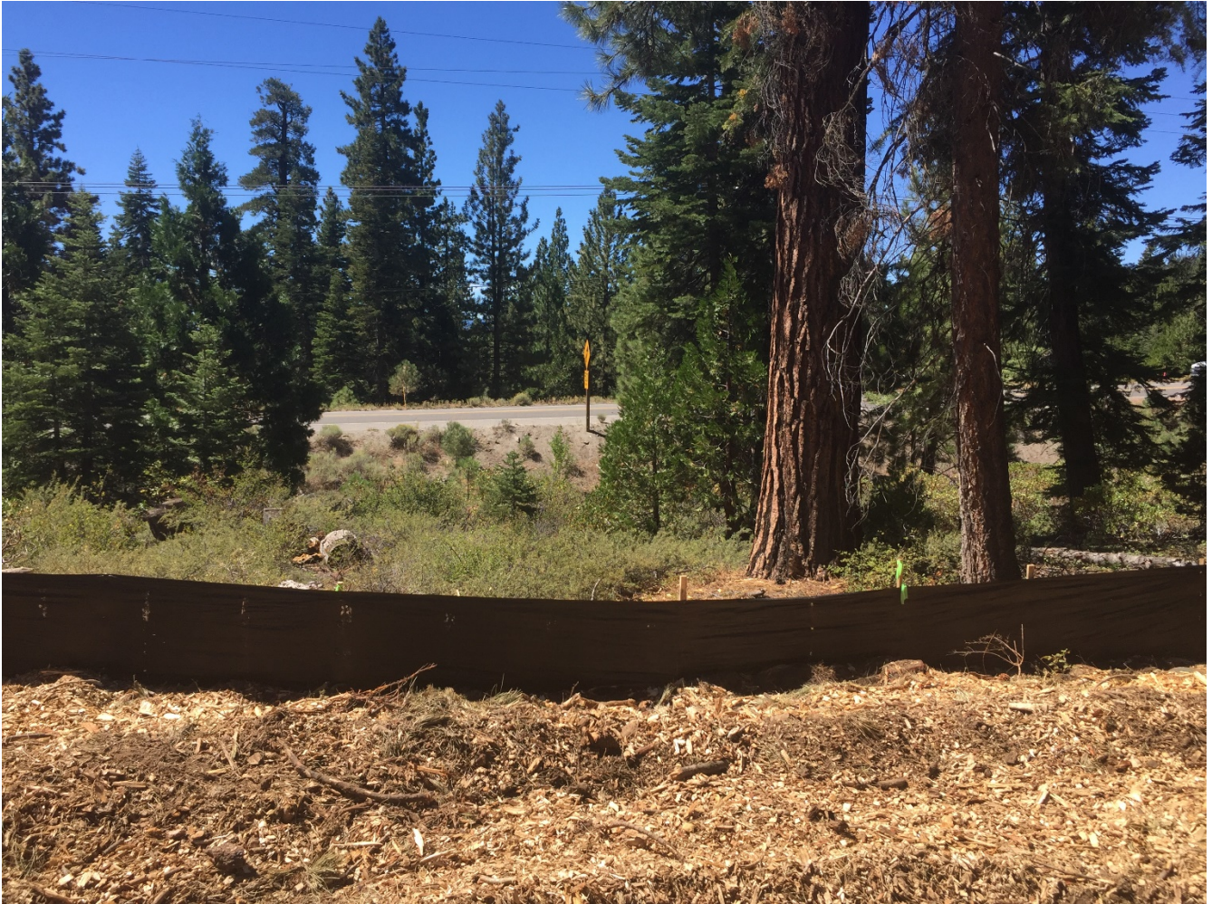
Photo 2: BMPs (silt fence) installed between ROW and Highway 267 (APM-SOILS-1).
