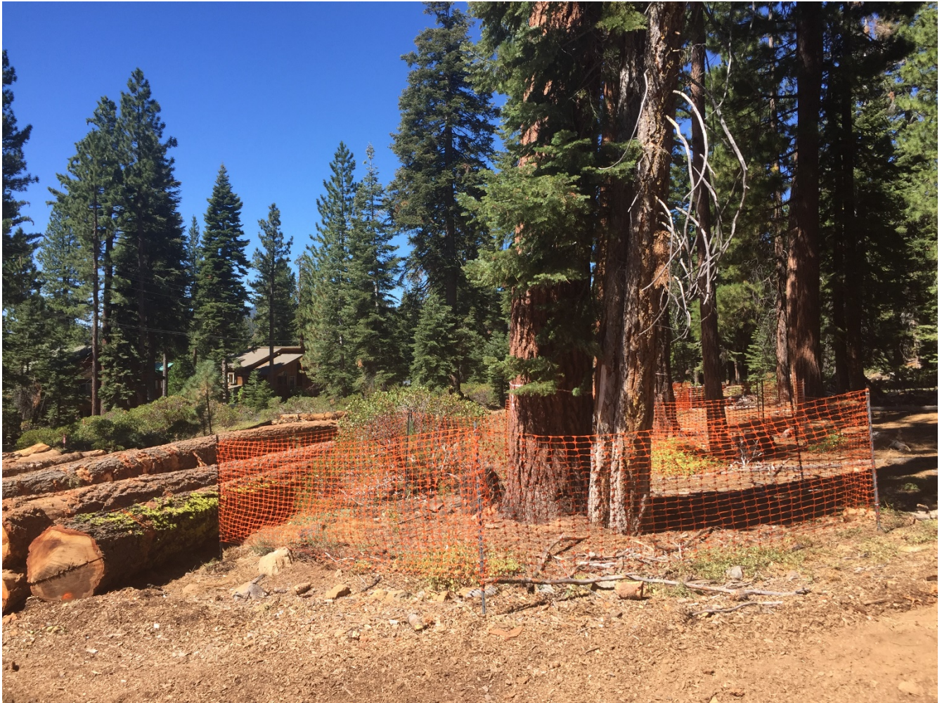
Photo 3: Tree protection fencing installed within Lake Tahoe Basin.
