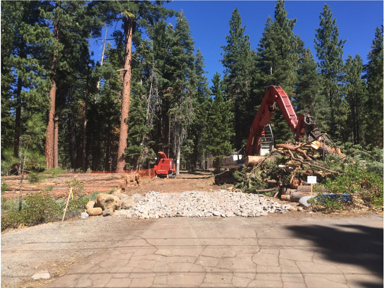
Photo 6: Project access with stabilized entrance, in compliance with APM-AQ-8.
