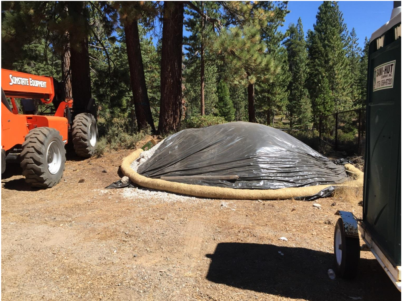
Photo 2: Soil stockpiles covered (APM-AQ-6).
