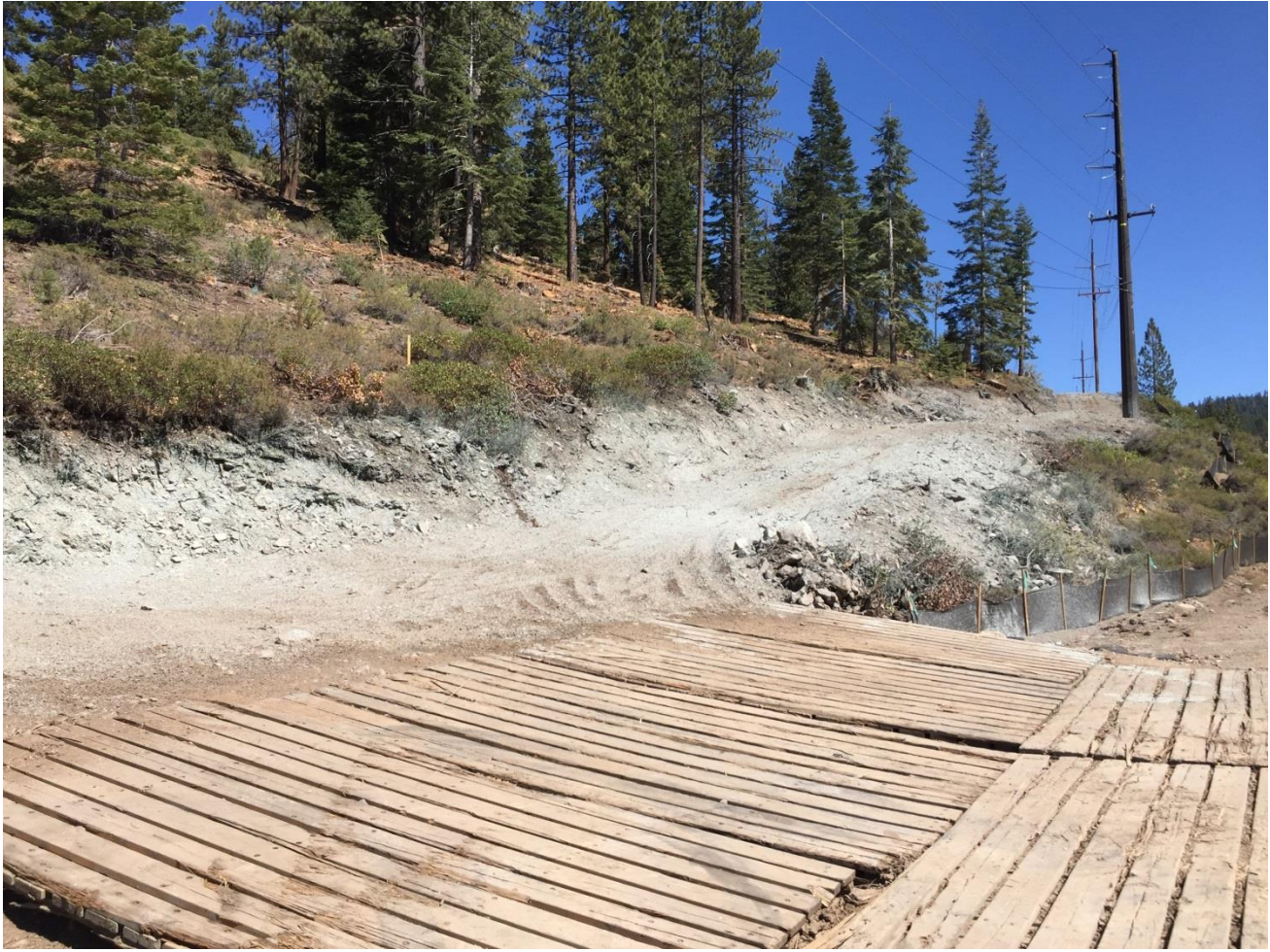
Photo 4: ROW hydroseeded, temporary matting installed to facilitate access and minimize soil disturbance.
