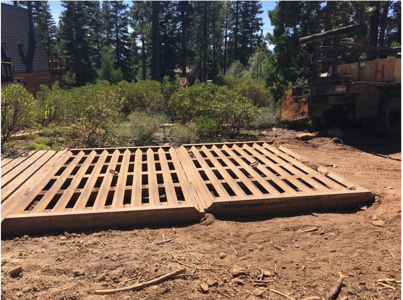
Photo 3: Stabilized ROW entrance to minimize track-out onto public roads (APM-AQ-6).
