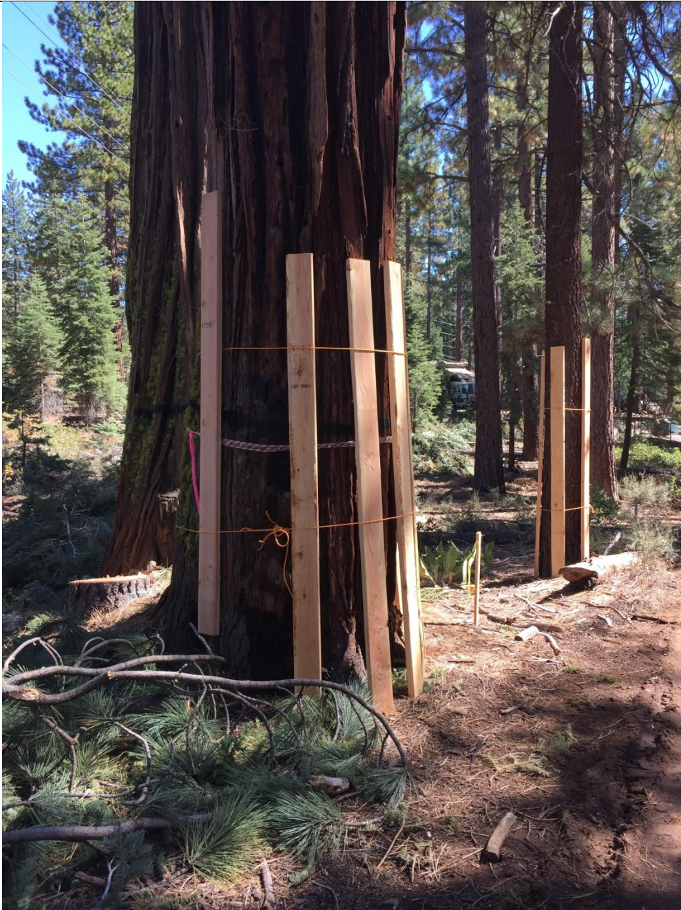
Photo 5: Temporary retained tree protection measures, near Kings Beach Substation.
