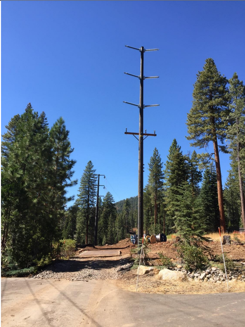
Photo 6: New pole installed (#291213) and stabilized entrance, in compliance with APM-AQ-8.
