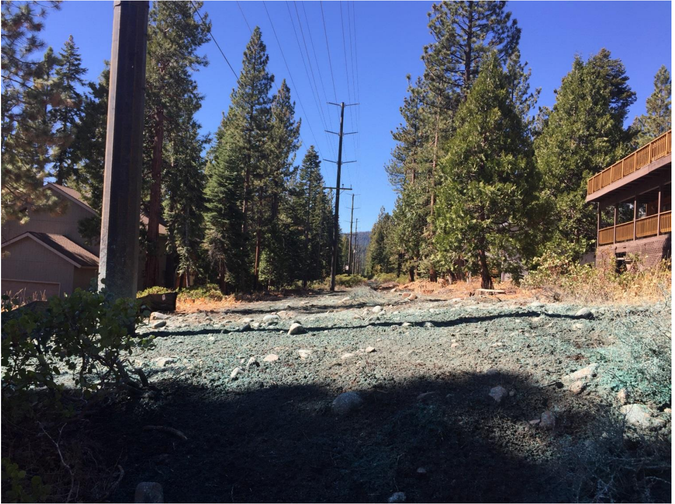
Photo 2: Project right-of-way near Pole 291223, hydroseeded.
