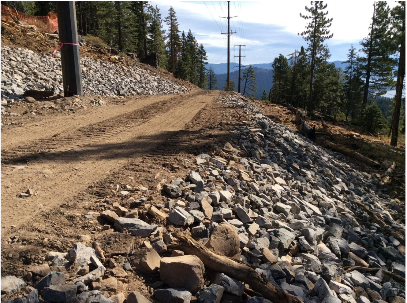
Photo 5: Right-of-way on U.S. Forest Service property, temporary BMPs still in place.
