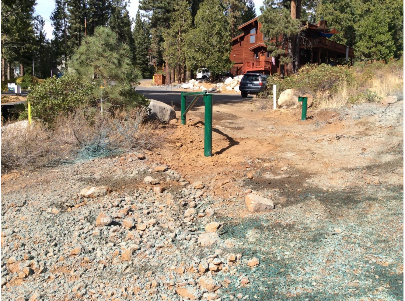
Photo 6: Right-of-way hydroseeded and access control gate installed at end of Canterbury Drive.
