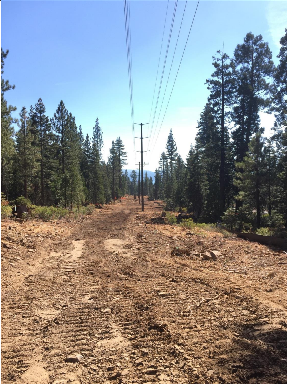
Photo 1: Permanent access road graded, restoration not yet complete.
