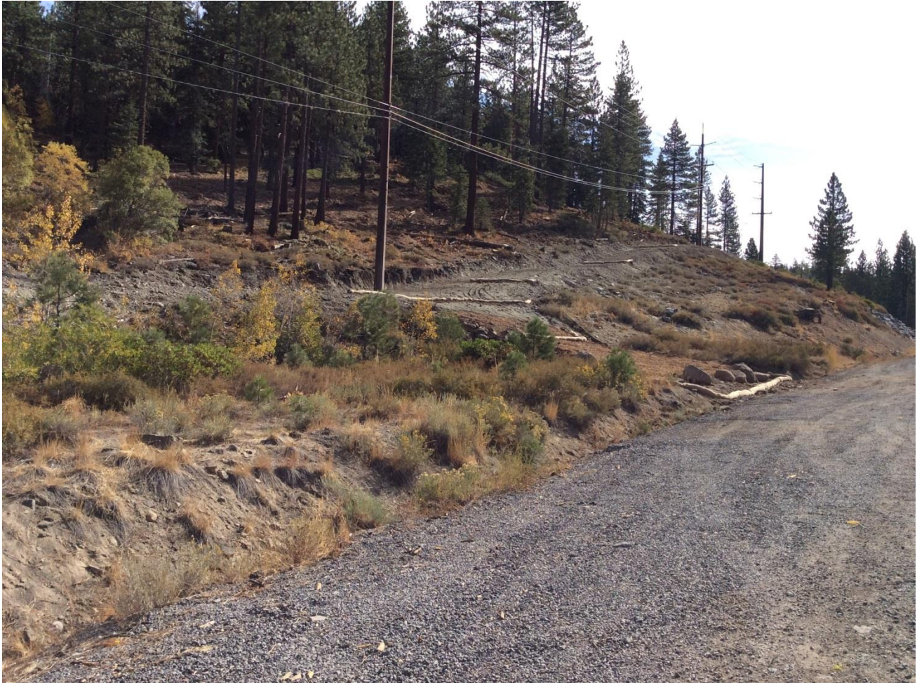
Photo 4: Right-of-way access point along Highway 267 with much, hydroseed, and wattles installed.
