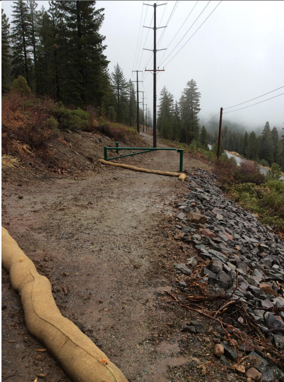
Photo 4: Right-of-way access gate installed on U.S. Forest Service property.
