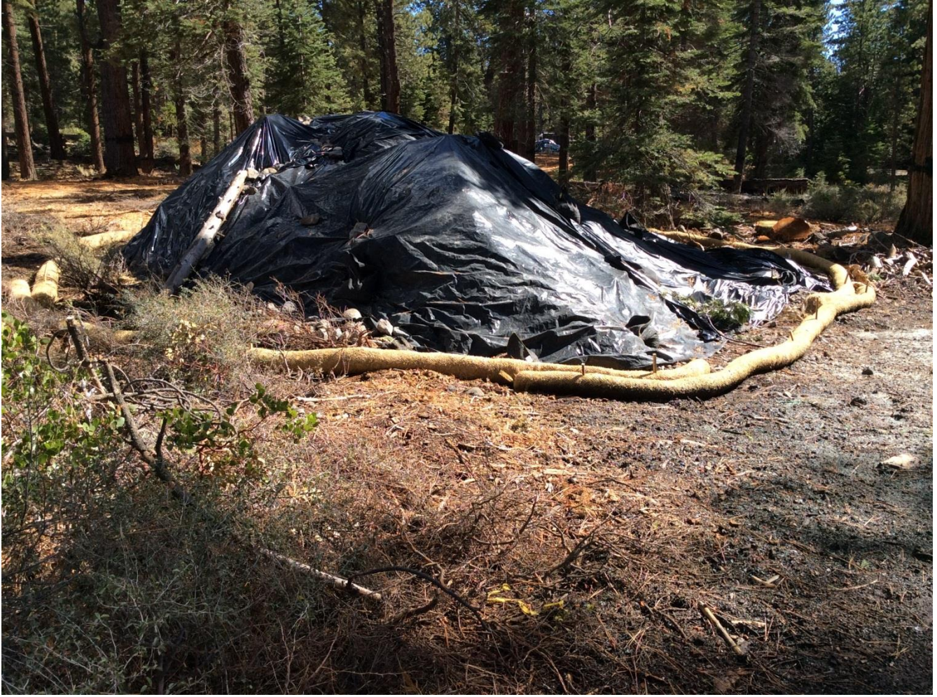
Photo 1: Soil stockpile near Kings Beach Substation covered for winter.
