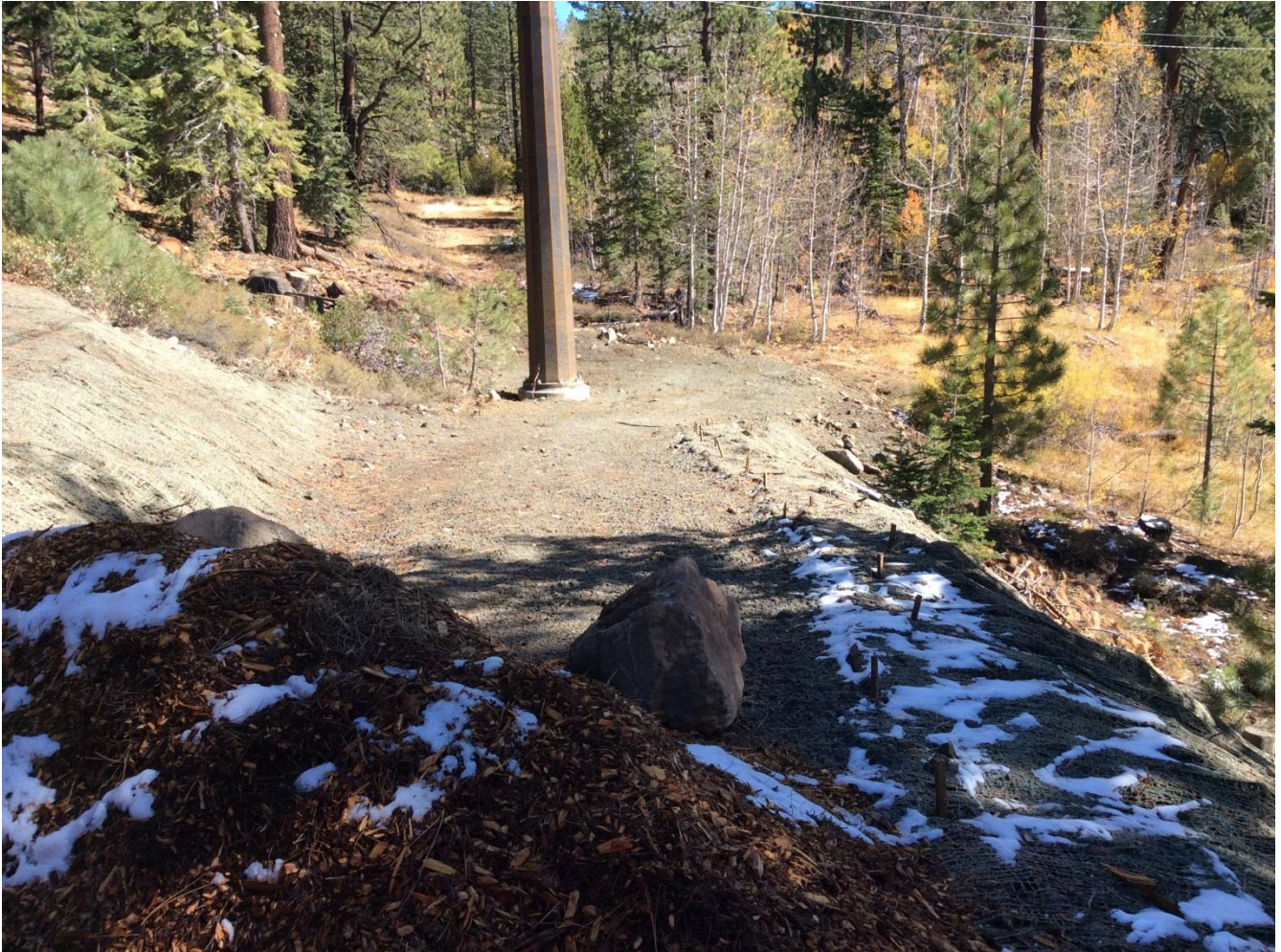
Photo 2: Project right-of-way near Pole 291160 with access blocked (boulders) and BMPs installed.
