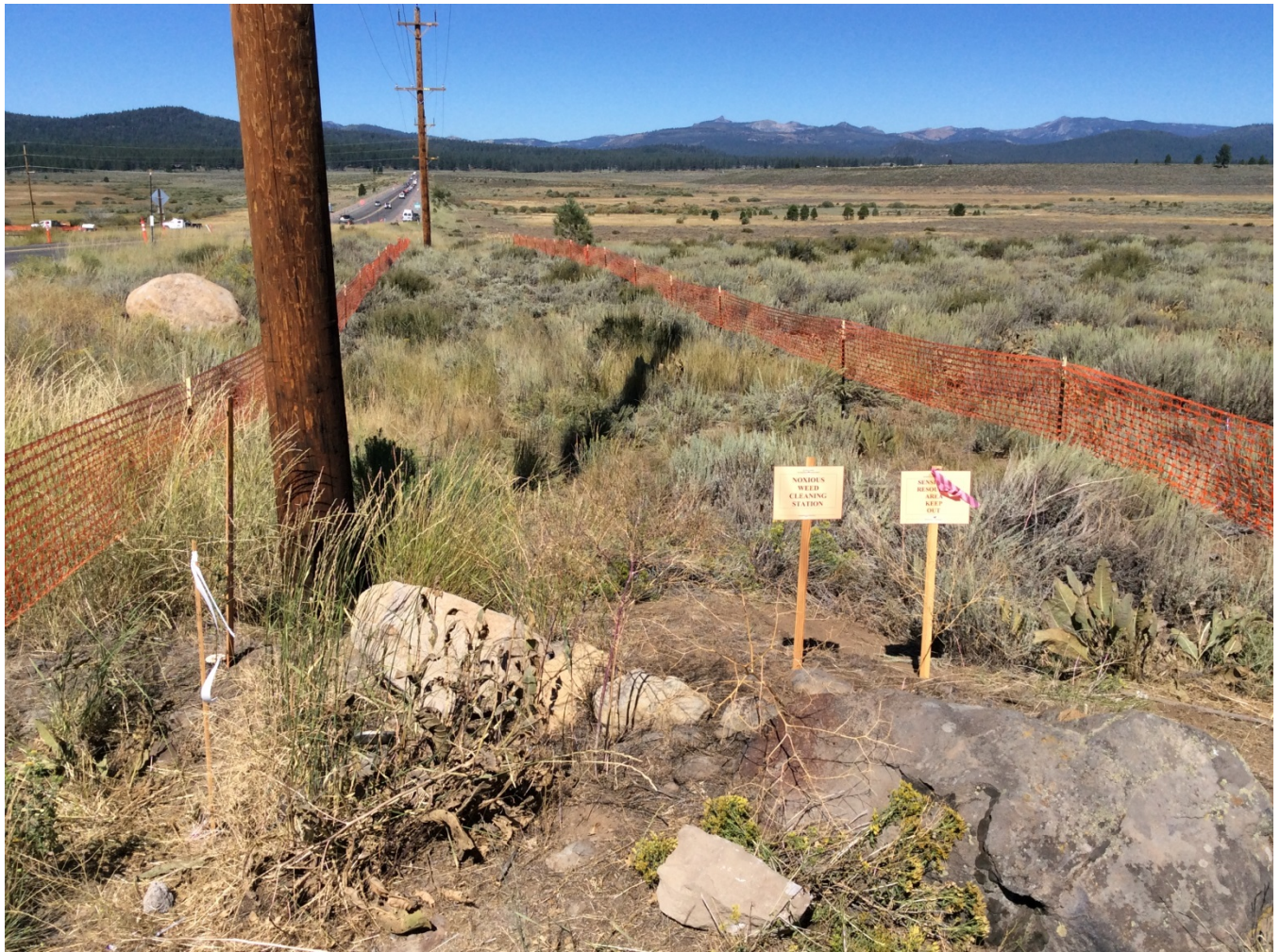
Photo 3: Fencing installed to delineate approved work areas and sign indicating sensitive resource exclusion area, consistent with APM-BIO-26 and the project's Flagging, Fencing, and Signage Plan. Second sign identifies noxious weed cleaning station, consistent with APM-BIO-5.
