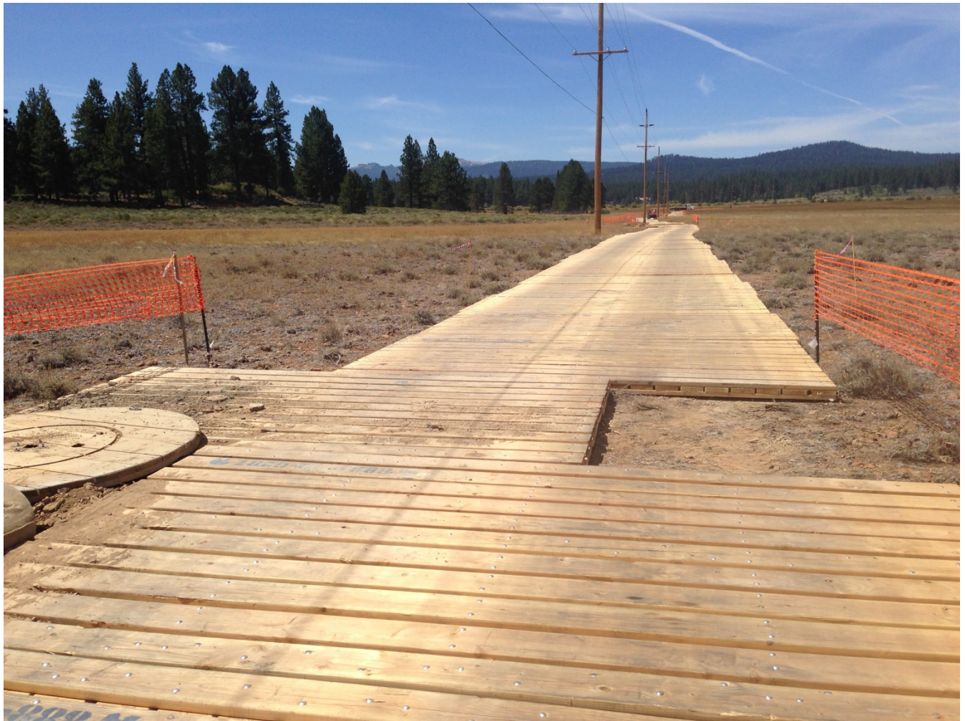
Photo 4: Timber matting in Martis Valley shifted onto open excavations, resulting in overland travel in upland areas. Liberty Utilities stated they will use other materials to cover excavations, which will be confirmed in subsequent compliance inspections.
